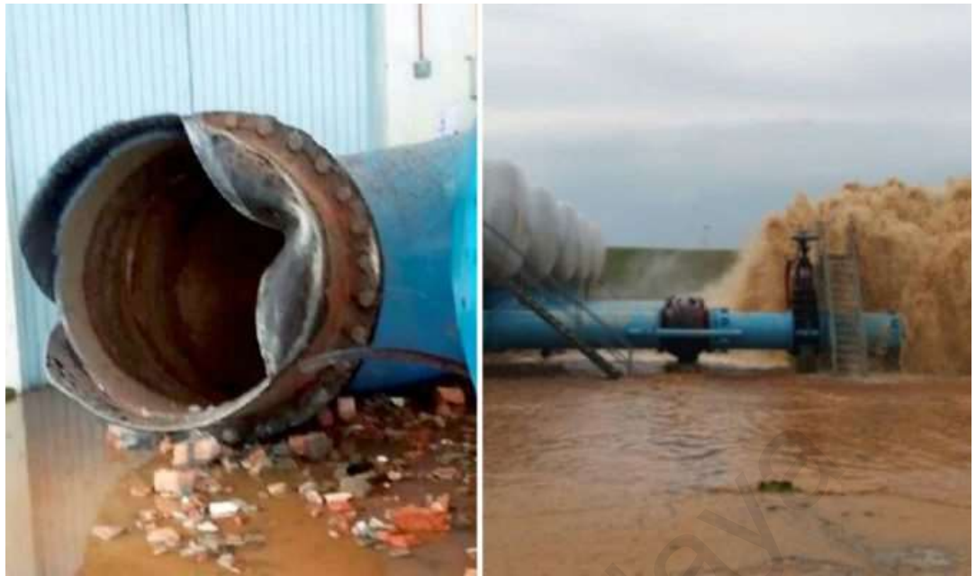
Figure 1.1: Pipe burst cause of water hammer
