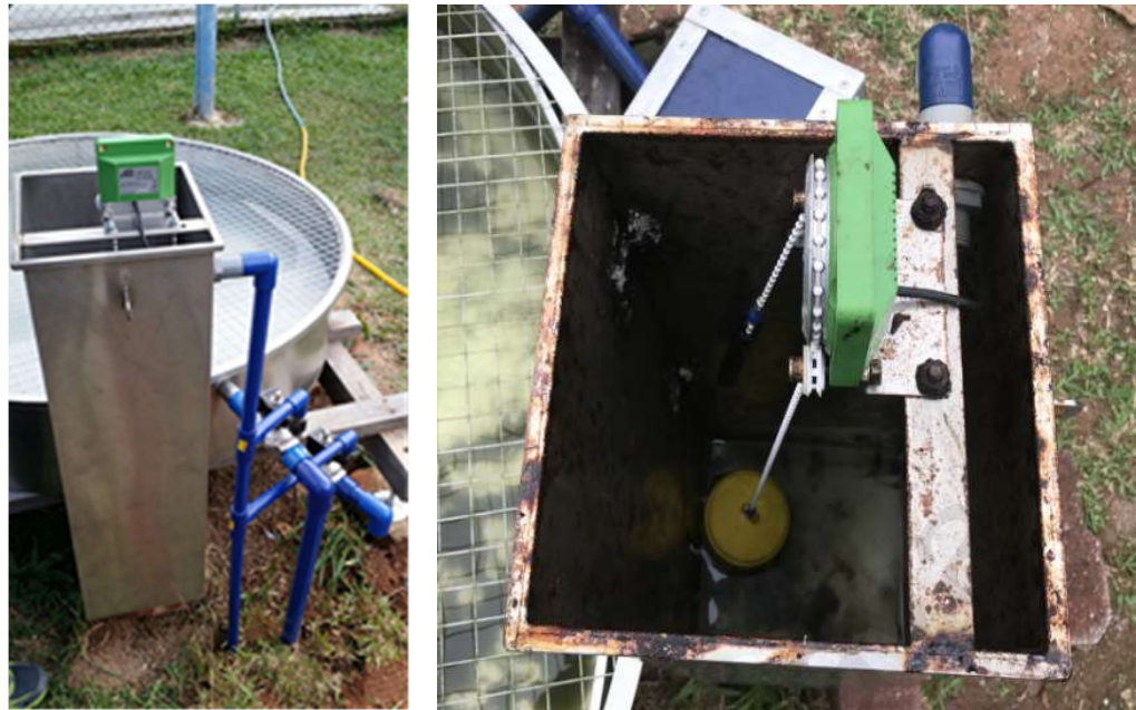
Figure 2.14: The shaft encoder water level sensor on top of the stilling well
