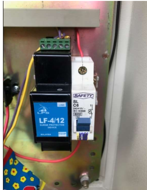
Figure 2.24: Surge protection device
