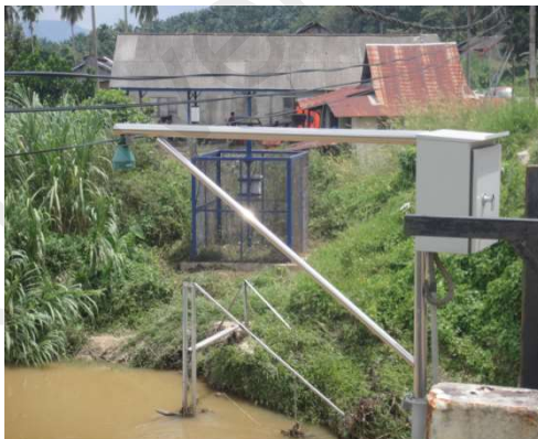
Figure 3.4: Ultrasonic water level sensor
