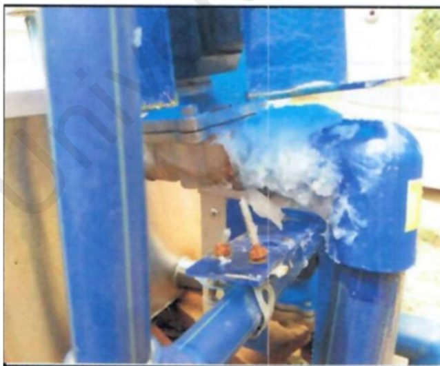
Figure 3.14: Leaking at the valve joint
