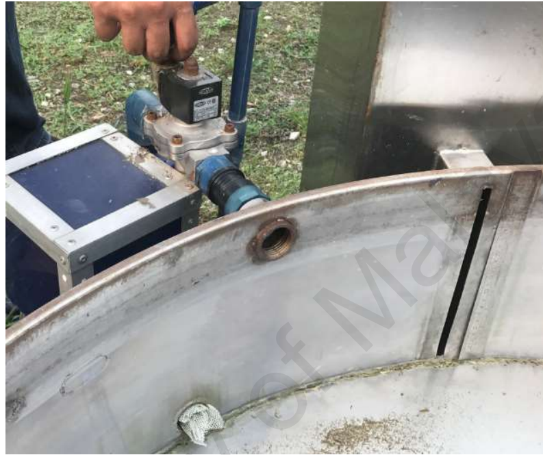
Figure 2.18: Solenoid valve installed at site
