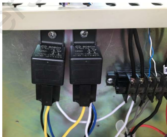
Figure 2.19: The connected 12V relays inside the enclosure
