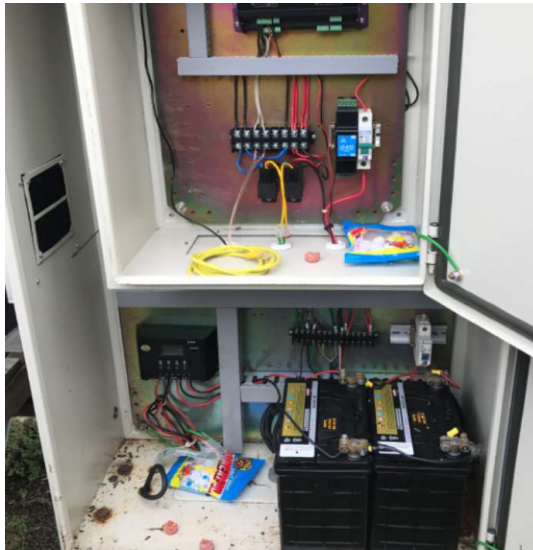
Figure 2.25: Battery and solar charge controller
