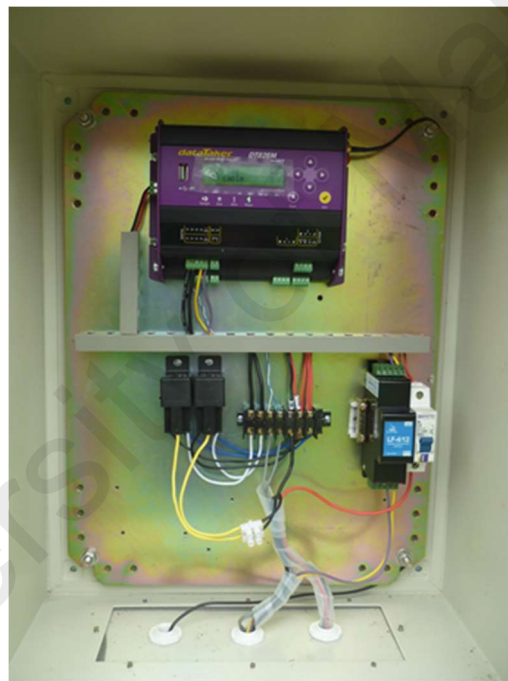
Figure 2.17: Datalogger RTU inside the enclosure
