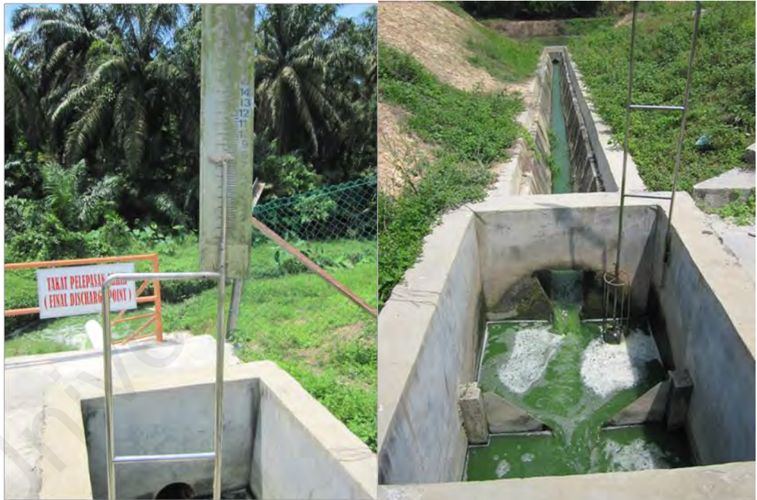
Figure 3.29: Final discharge point of treated effluent to waterbody and subjected to Environmental Quality Regulations 1978
