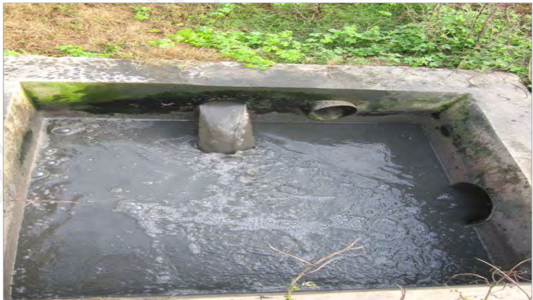
Figure 3.27: Raw effluent after passing the rubber trap and before entering the anaerobic pond
