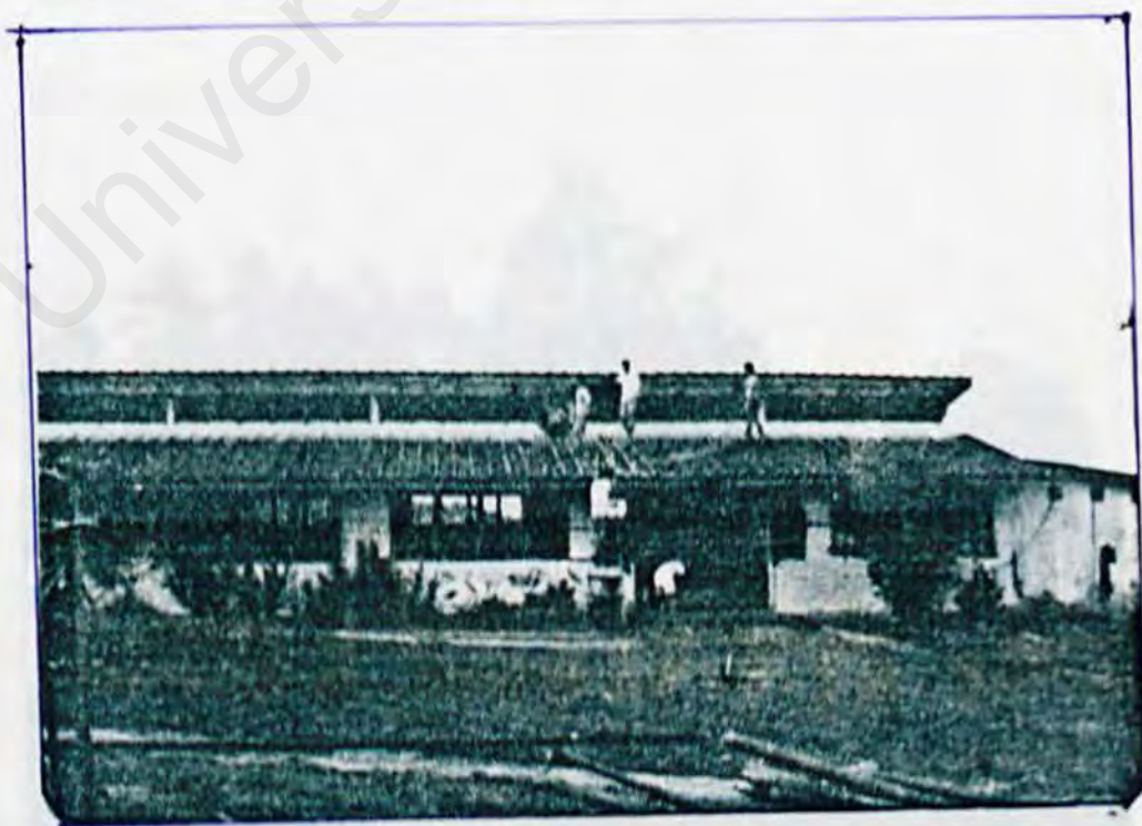
Plate 6 : Maintenance crew at work, repairing the roof of Tunas Baru
