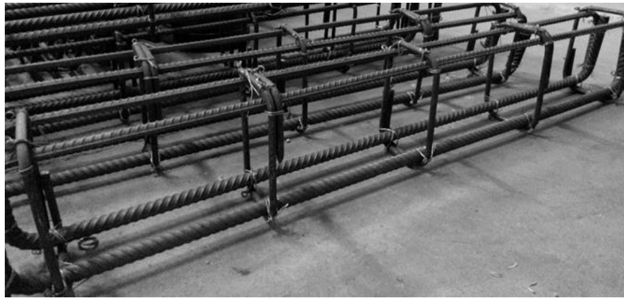
(a) steel reinforcements
