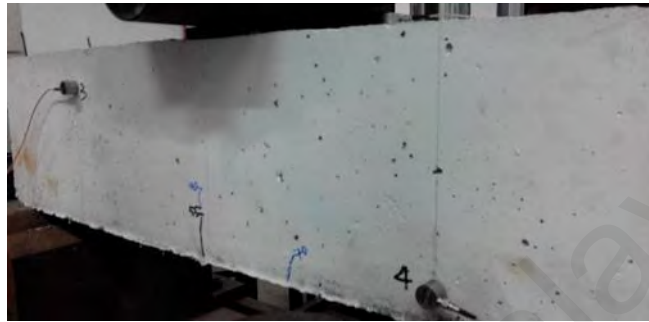
(a) First visible crack
