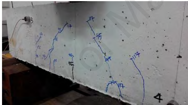
(b) Cracks distribution
