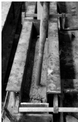
(b) casting of beam
