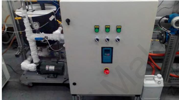
**Figure 3.17:** Photograph of the controlling unit that attached with SCADA system.
