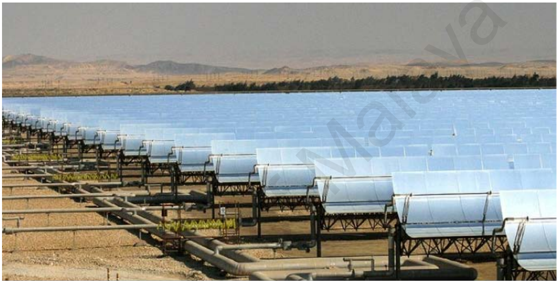
Figure 2.6: Row of PTC arranged in parallel
