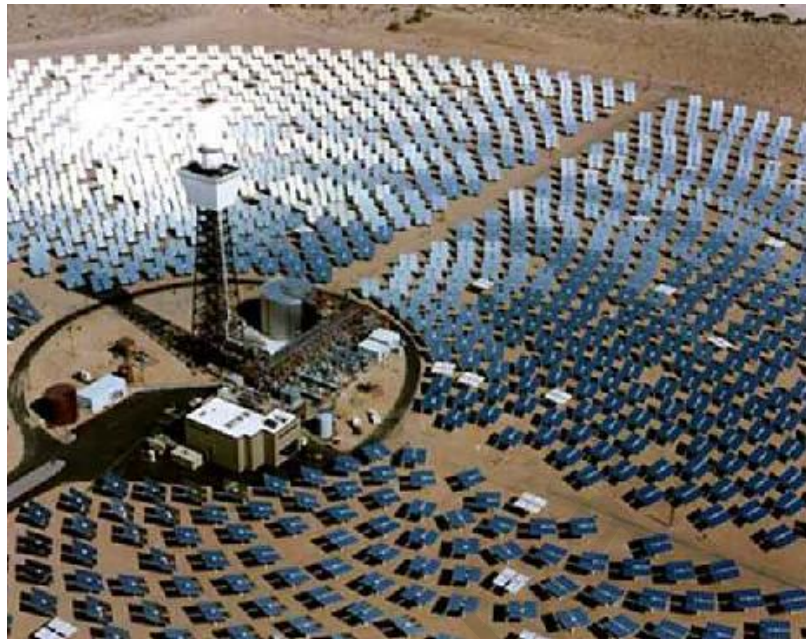
Figure 2.9: Heliostat array located in California
