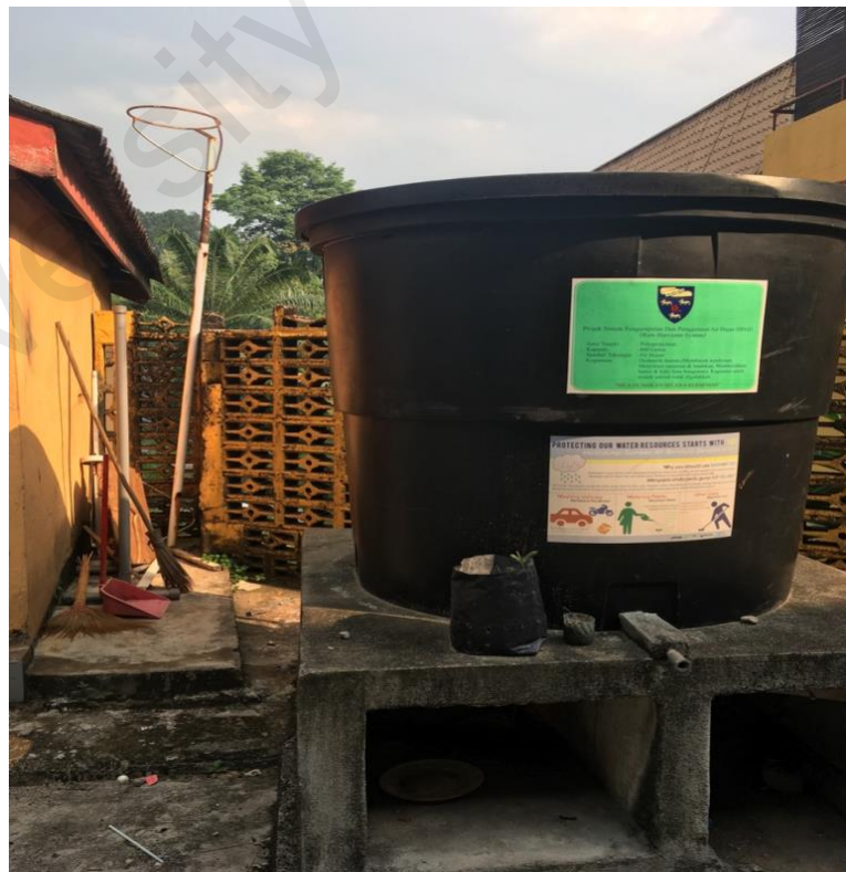
Figure 4.1.2 (b) Missing pipe and unusable tank at Kinabalu Residential College
