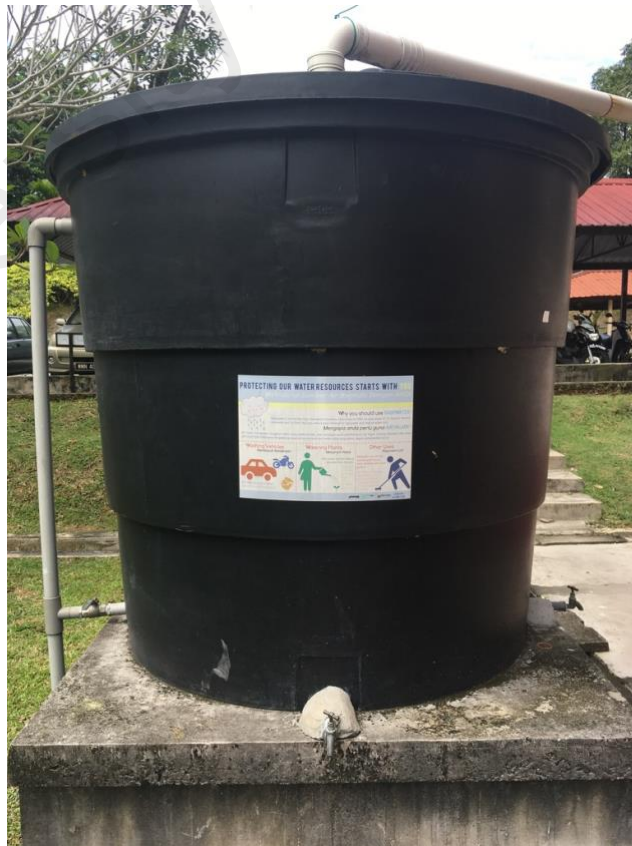
Figure 4.1.1(d) Good condition of RWHS tank
