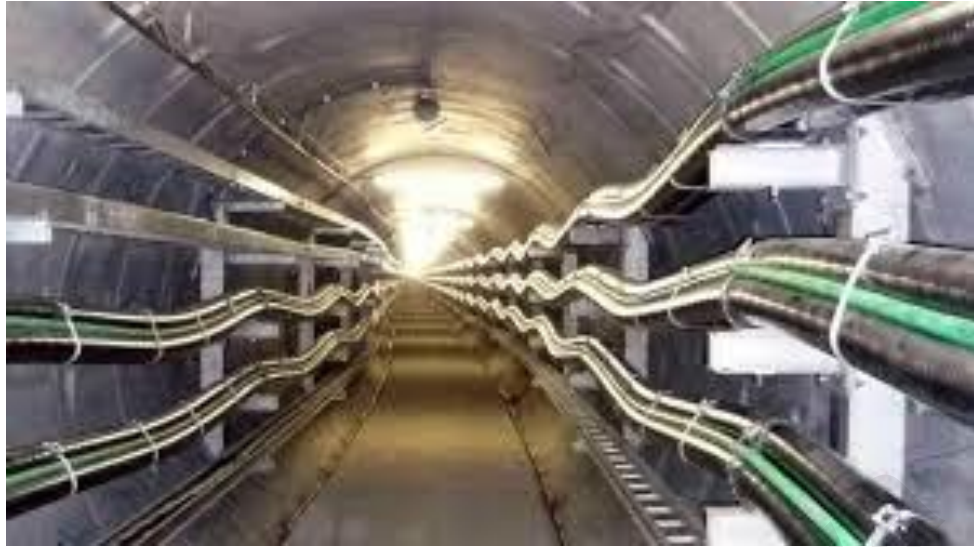
Figure 1.1: Utility tunnel, ( http: https://www.ancon.co.uk )
