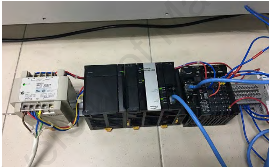
Figure 5.8: Omron NJ101-1020 machine automation controller powered on by Omron S82K-05024 power supply, serves as the operation center in the test rig.
