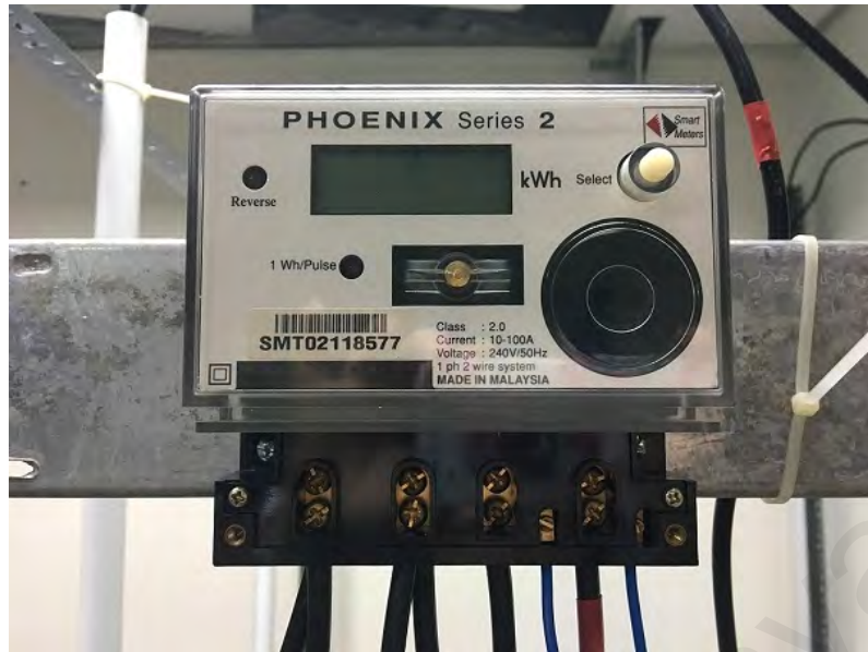
Figure 5.7: The Phoenix Series 2 smart meter.
