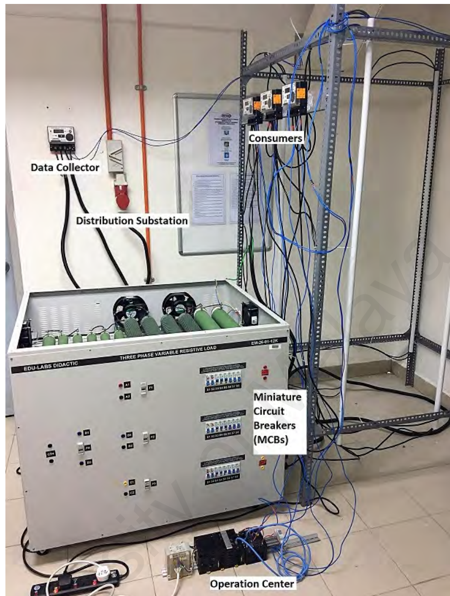
Figure 5.4: The hardware experimentation of the AMI test rig.
