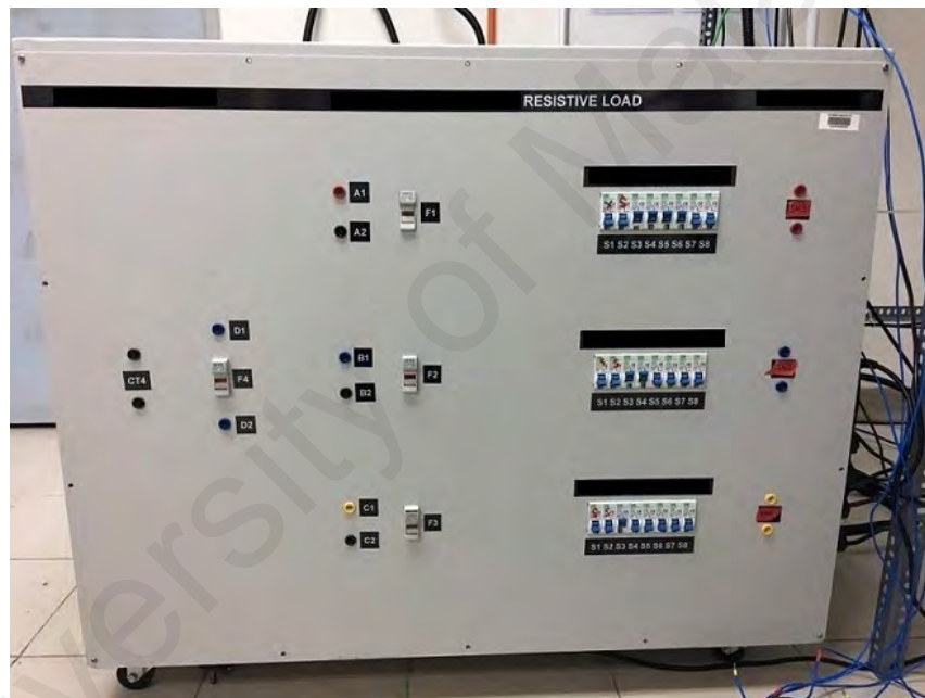
Figure 5.12: Miniature circuit breakers are attached to a metal plate at the front part of the load bank to prevent electrical shock.
