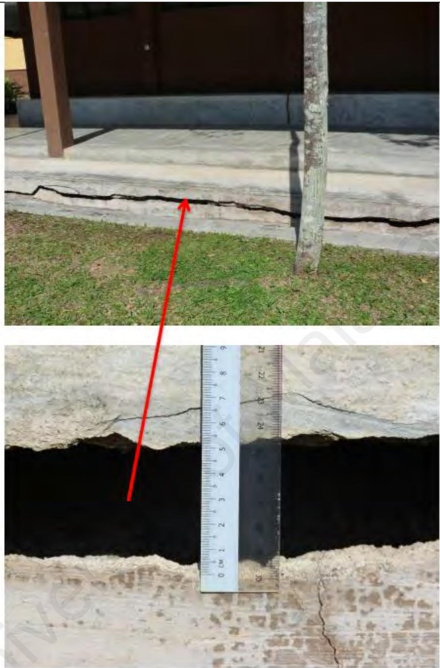
**Figure 3.3:** The visual observation of elongated cracks in SMK site.
