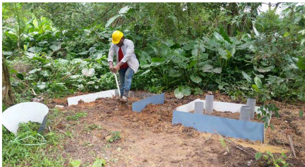
Plate 3.3: Construction of barrier to minimize leachate flowing into the experimental plot
