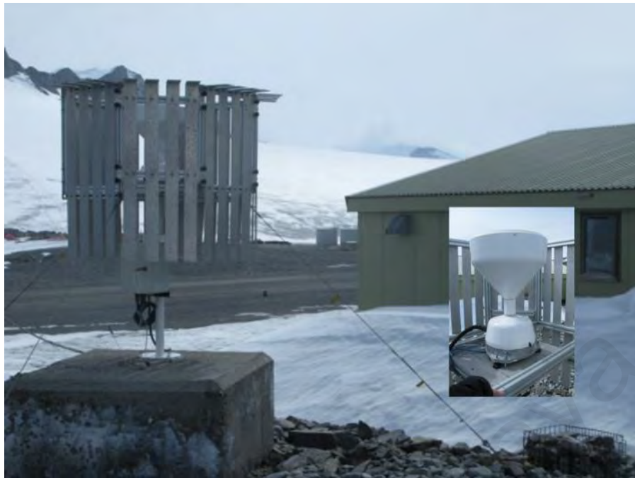
Figure 3.2 The UPG-1000 system installed at Rothera.
