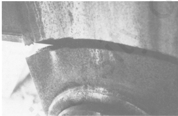
a) Anchorage plate failure of the support at the East abutment
