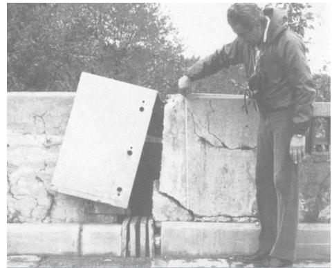
b) Damage to concrete cover at the West abutment
