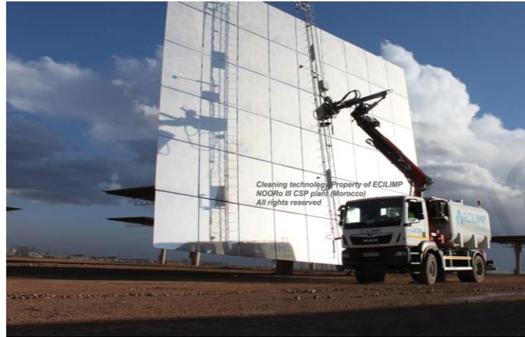
Figure 2.20: Semi-automatic cleaning of heliostats in Noor III (Bouaddi et al., 2018)
