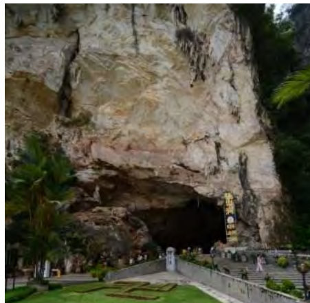
Figure 4.59: Location of KLT 1 (c) which located exactly above the cave entrance.
