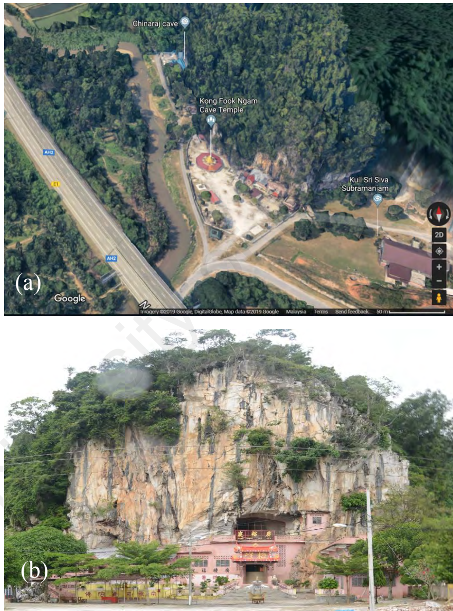
Figure 4.103: (a) Location of Gunung Lanno limestone hills (b) Gunung Lanno rock slope for stability analysis.
