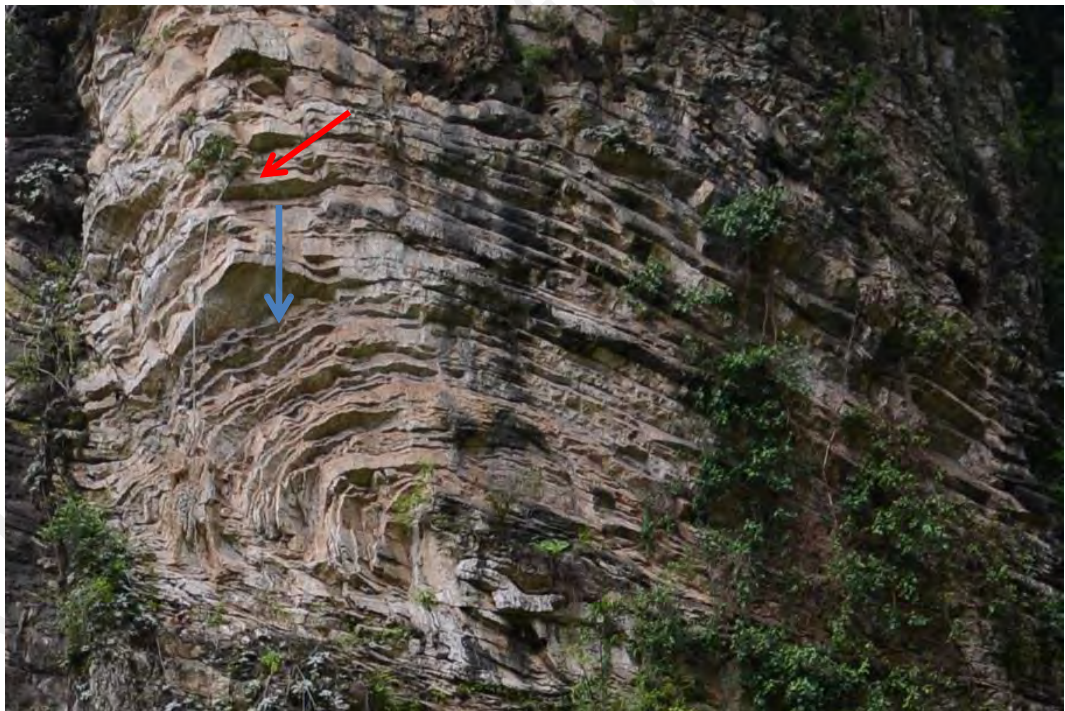
Figure 4.71: Example of possible planar failure involving J2 (80/100) in green point cloud view, Blue arrow represents the dip direction of J2 joints which is daylighting and is a potential for planar failure. Red arrow represents J1 (64/279) dipping direction which is dipping into the slope.
