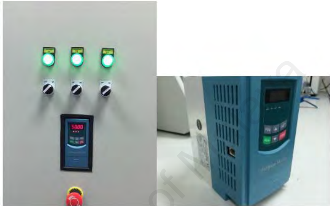
Figure 3. 9: Photograph of the Hoffman Muller inverter
