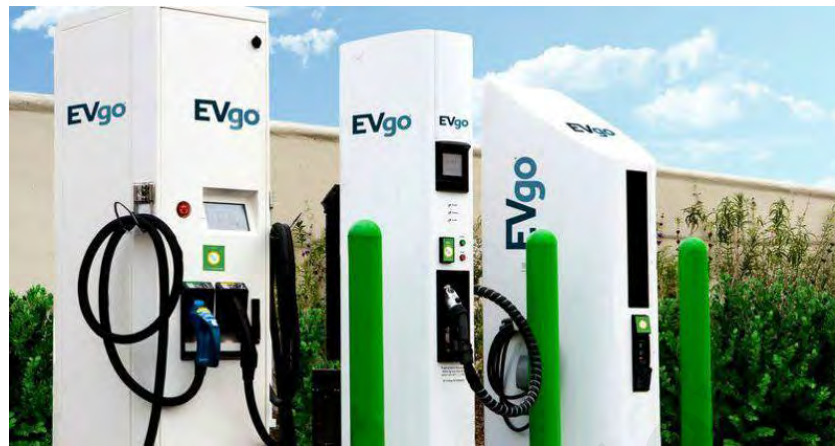
Figure 2.7: Charging station with DC fast chargers
