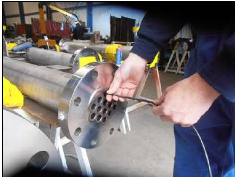
Figure 4.6: Example of Baroscopic Inspection
