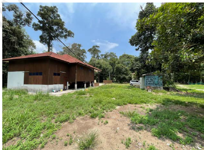
Figure 3.4: The back view of the building and this land is going to become the route of the water stream.
