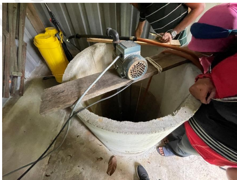
Figure 3.6: The existing borewell in the Rumah Hutan Jeram.
