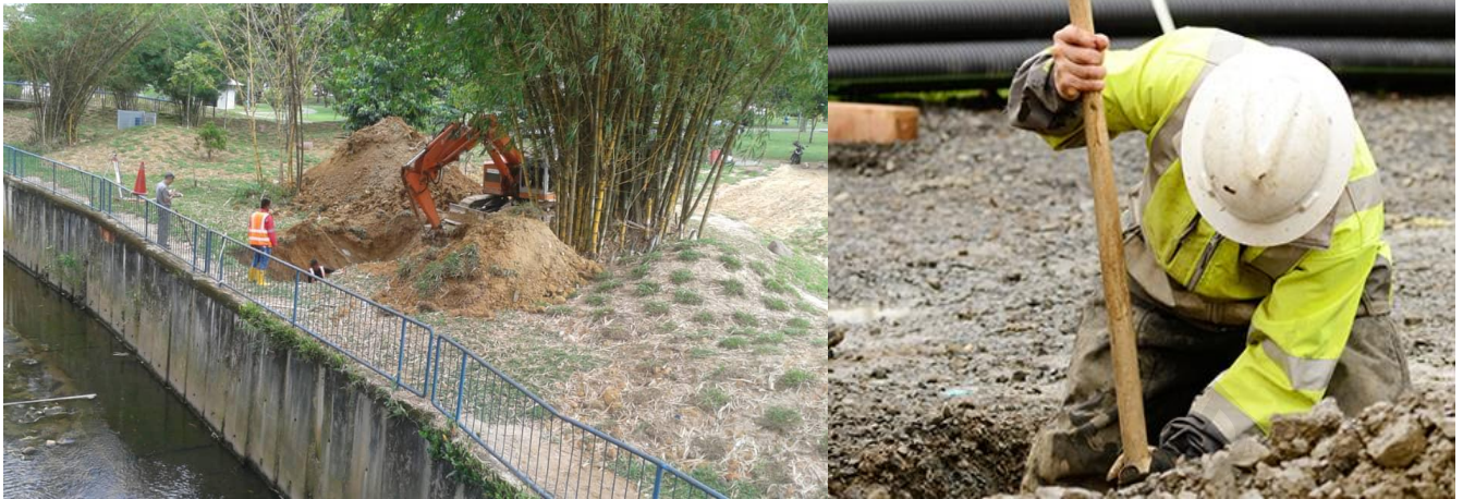
Figure 4.16 : Excavation and Manual Digging Activities
