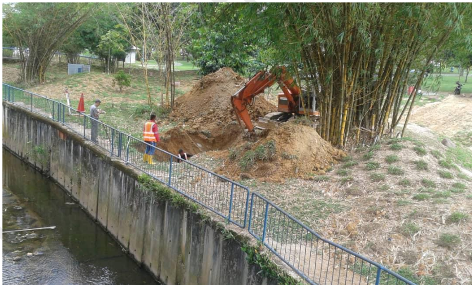
Figure 4.5 : Possible Cave in Hazards during excavation
