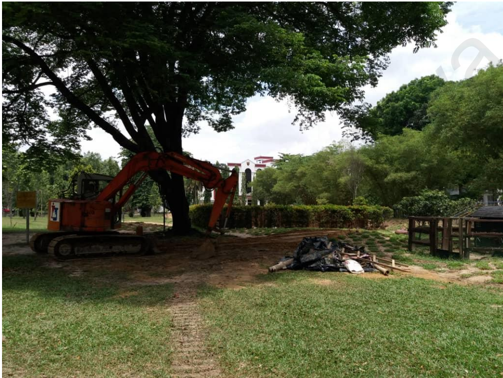
Figure 4.8 : Gathered construction wastes
