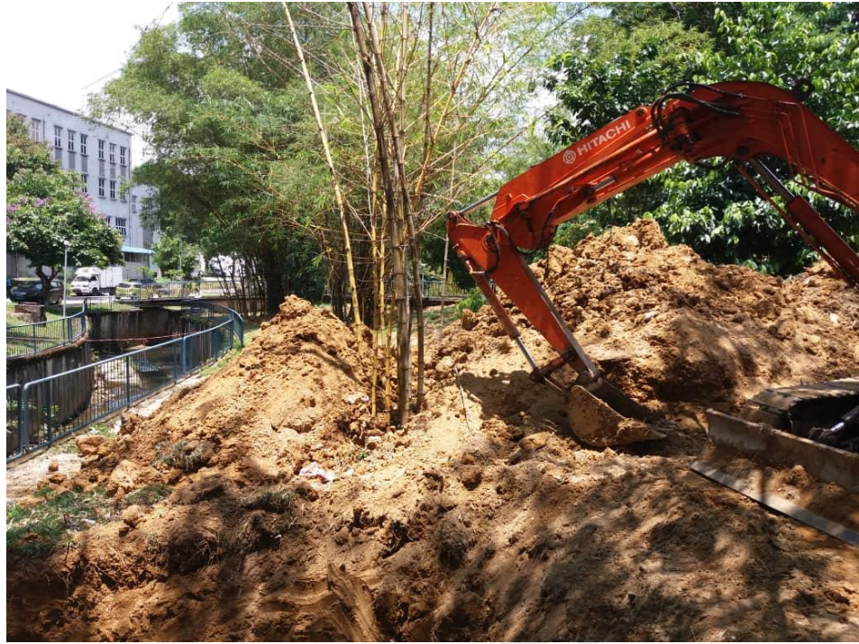
Figure 4.6 : Excavation during manmade wetland and streams construction
