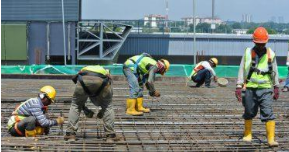
Figure 4.12 : Concrete Construction Activities
