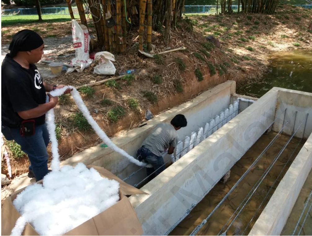
Figure 4.10 : Filtration Chamber Activities
