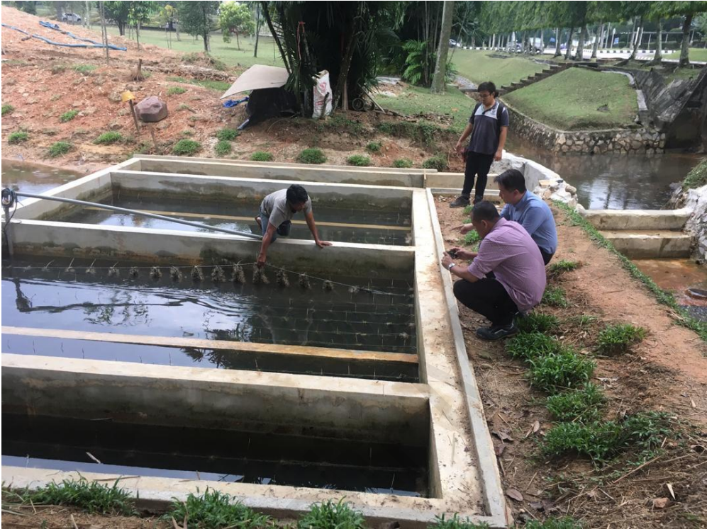
Figure 4.7 : Concrete Construction Activity
