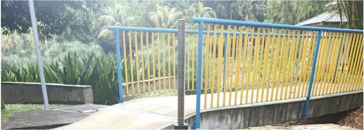
Figure 4.31 : Constructed Bridge near to Manmade wetland & streams
