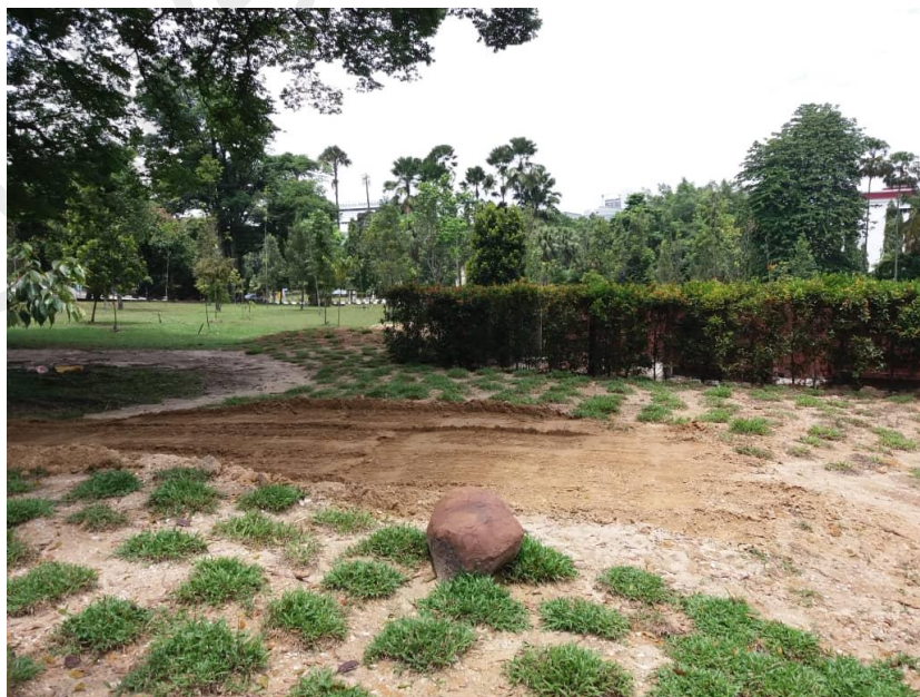
Figure 4.4 : Construction site for manmade wetland and streams
