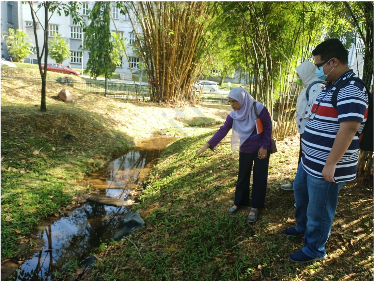
Figure 4.32 : Soil erosion and clear visibility of PET bags which were initially inside the soil
