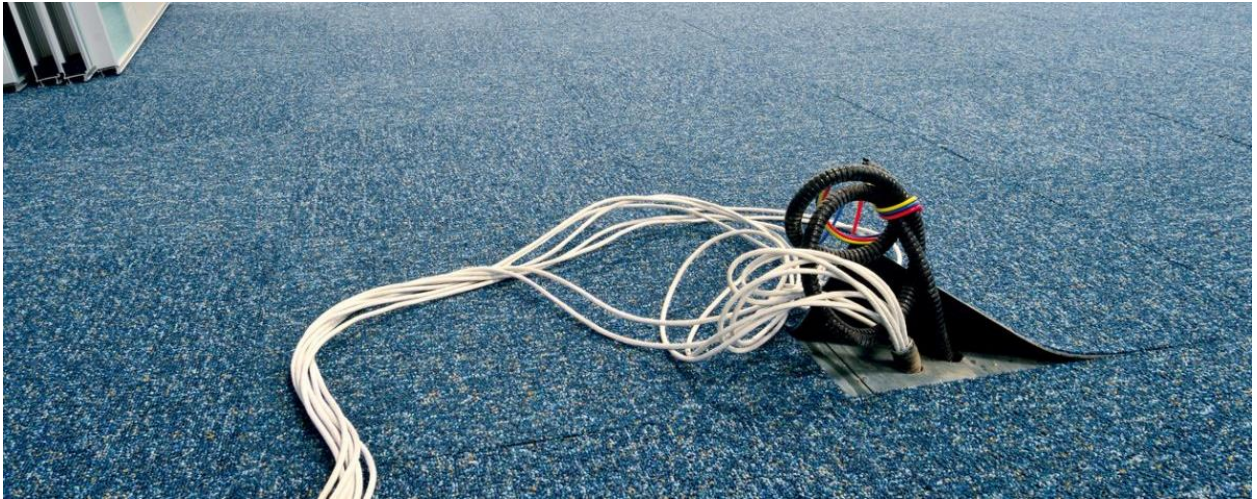
Figure 4.2: Example of cables left out on the floor.
