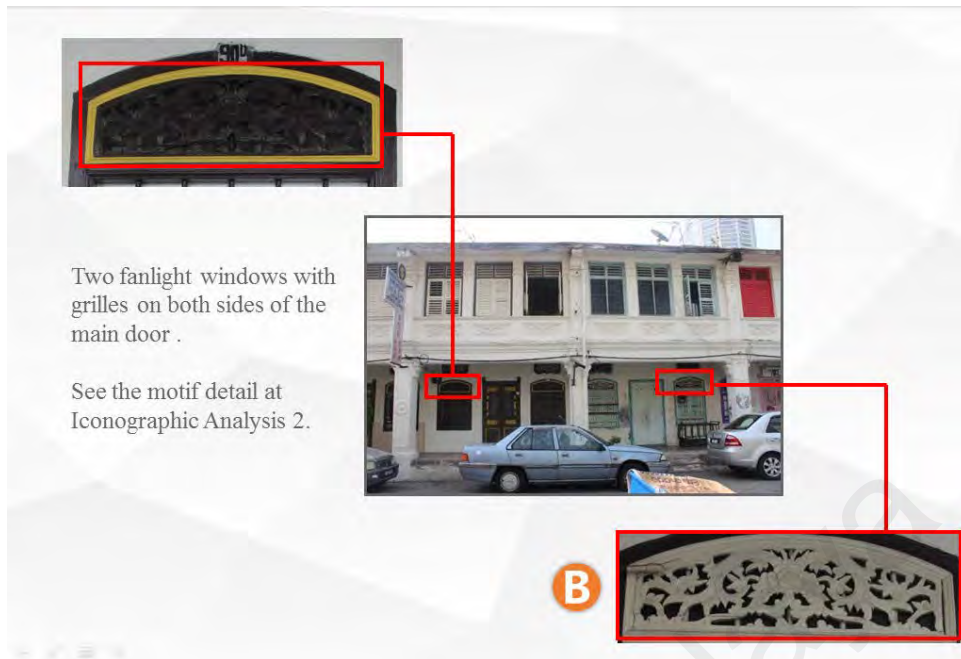
Figure 4.2: Two fanlight windows with wood carving grilles on both sides of the main door. Shophouse at Jalan Muntri. See the iconographic analysis at the following chapter. Photograph by Author.
