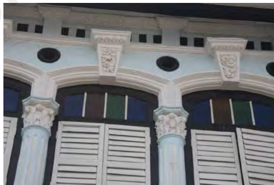
Figure 3.10: An applied ornamental on Penang Shophouse. Photograph: Author
