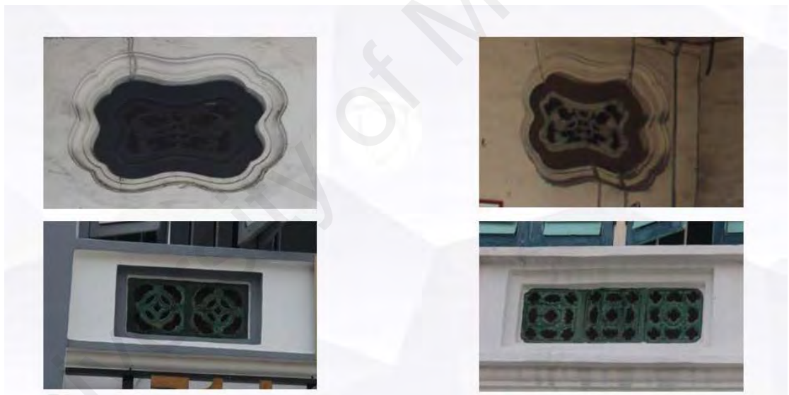
Figure 3.18: The different vents in ventilation function with ornament in woodcarving and ceramic. Photograph: Author
