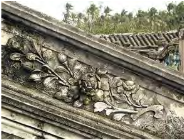
Figure 5.1: A motif on the roof ridge of traditional Hainan residential building.
