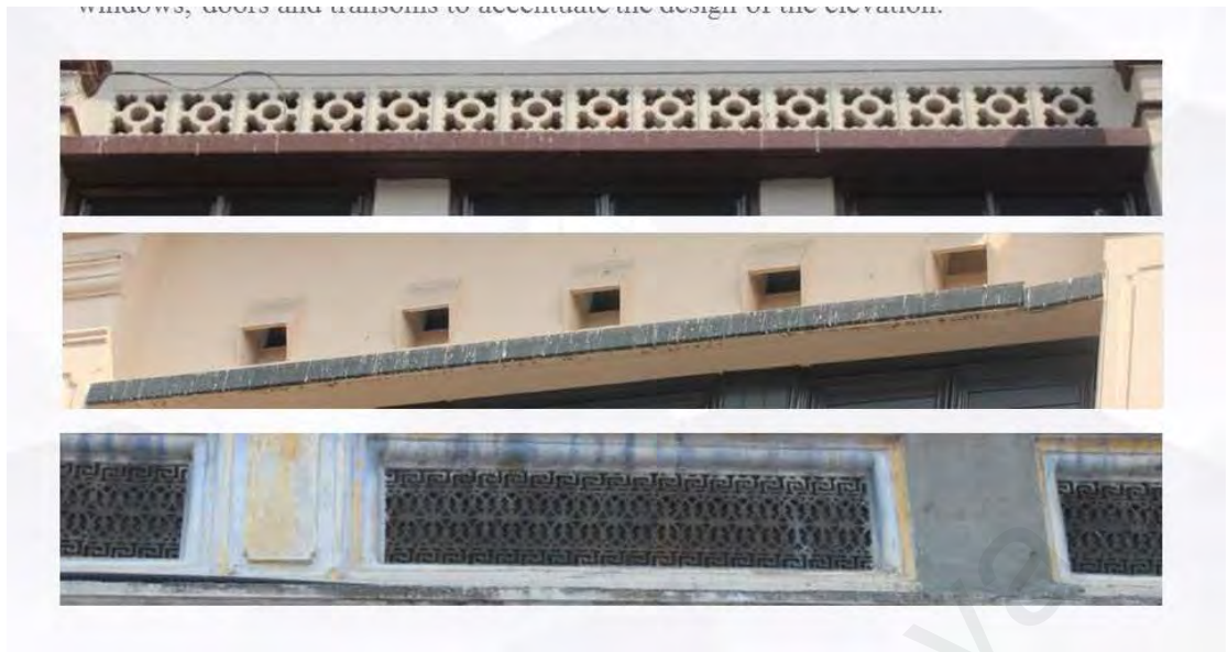
Figure 3.17: The different vents in ventilation function with simply ornament design. Photograph: Author
