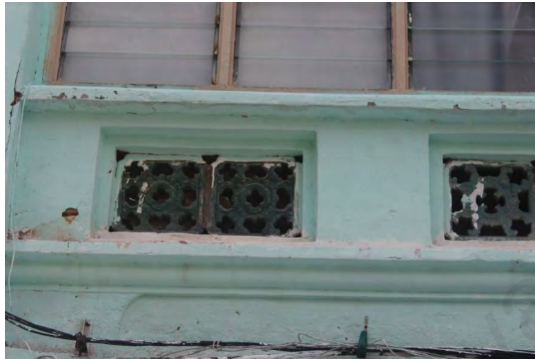
Figure 3.11: An organic ornament on Penang Shophouse. Photograph: Author
