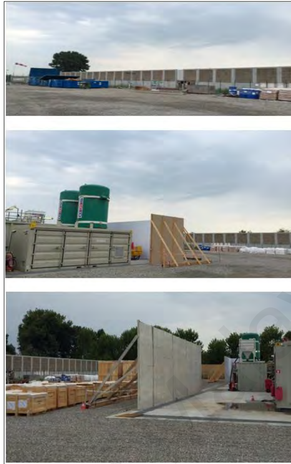
Figure 3.8: Noise barriers installed on Locations 1 and 2. Photographs by the author (2017).
