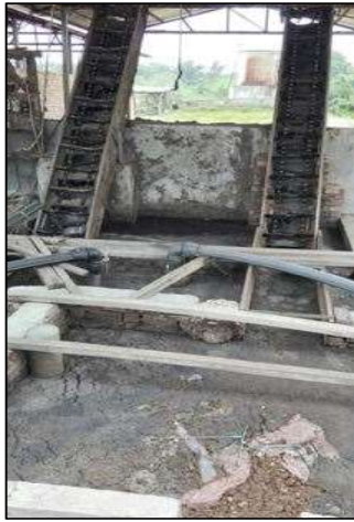
Figure 3.6: Decanter System at Pig Farm
