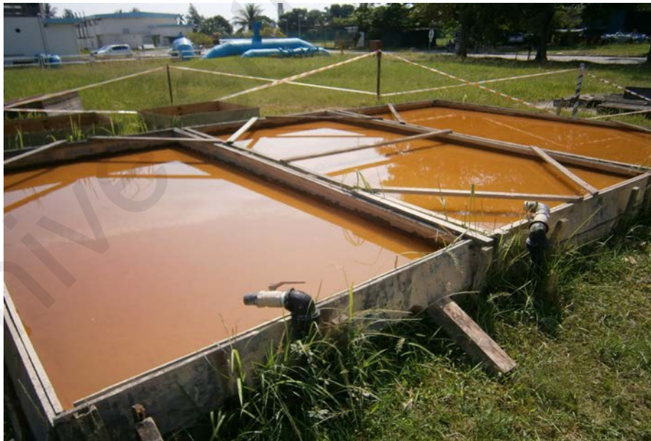
Figure 3.1: Water treatment residue pump from effluent discharge for drying.
