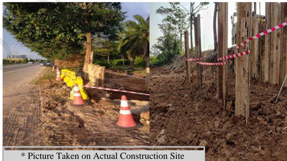
Figure 4.24: Sheet pile installed to prevent soil collision with warning tape.
