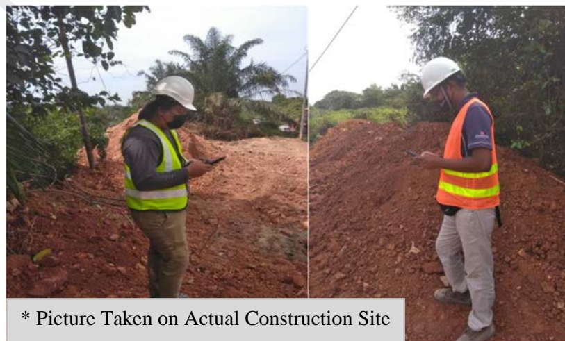
Figure 3.2: Construction personnel answering survey questionnaire.
