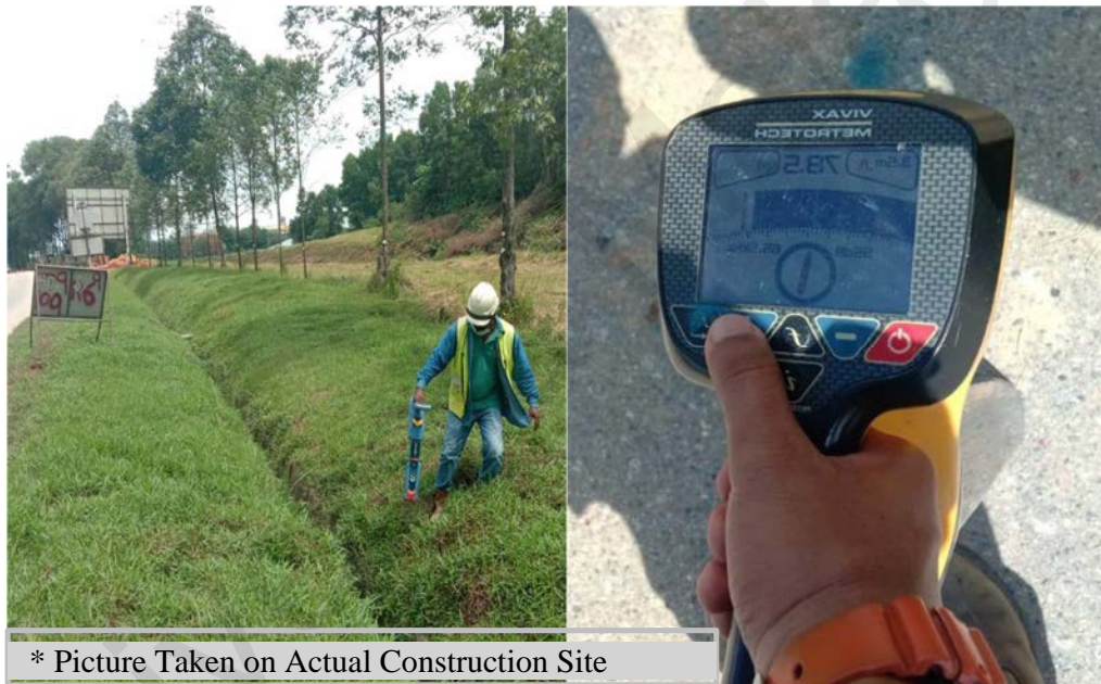
Figure 4.22: Underground utility detection before excavation works.
