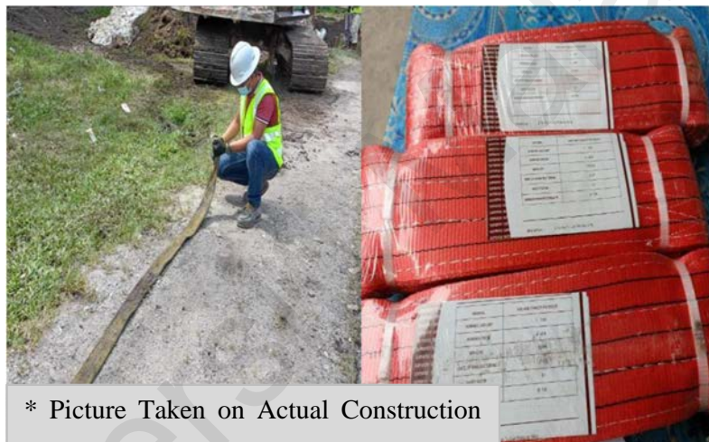
Figure 4.20: Lifting belt inspection and new belt standby onsite.
