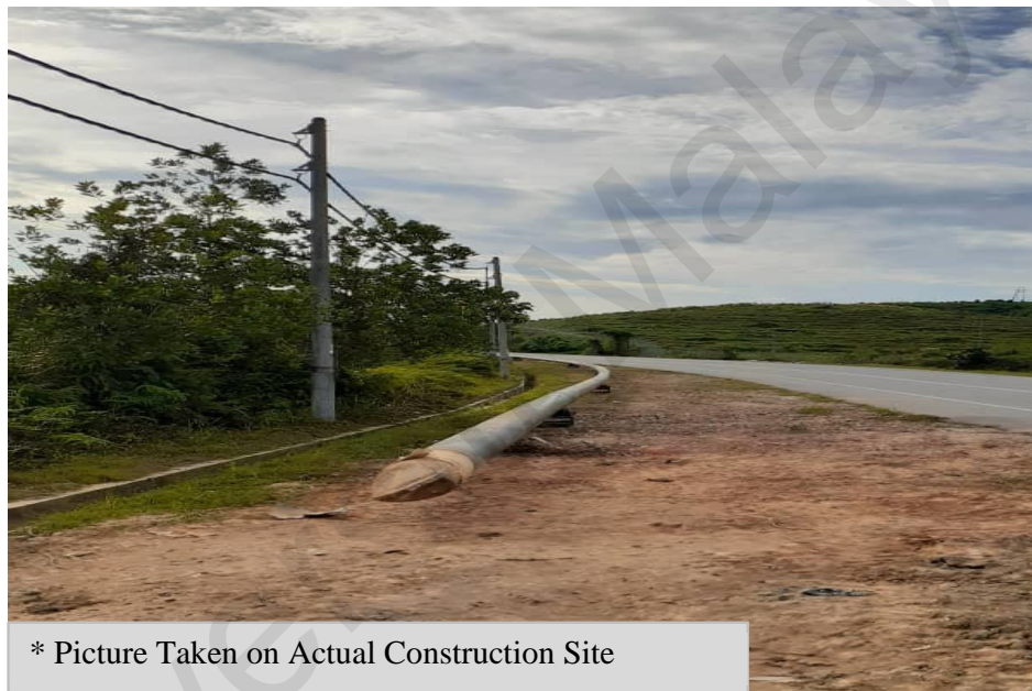
Figure 4.26: Pipe placed on roller ready for pulling process.
