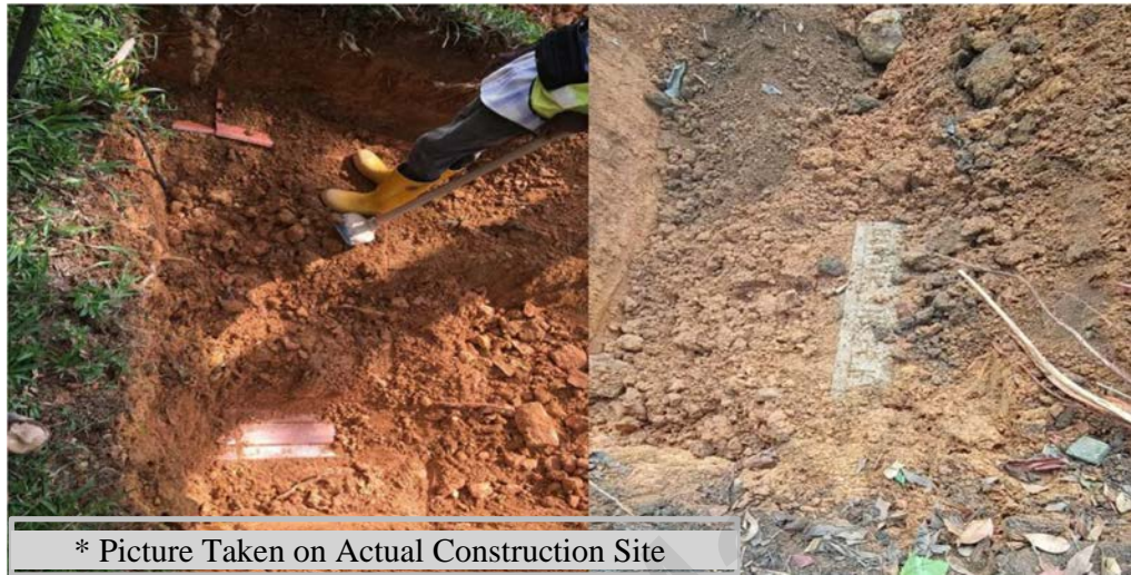
Figure 4.23: Existing utilities indication slab.
