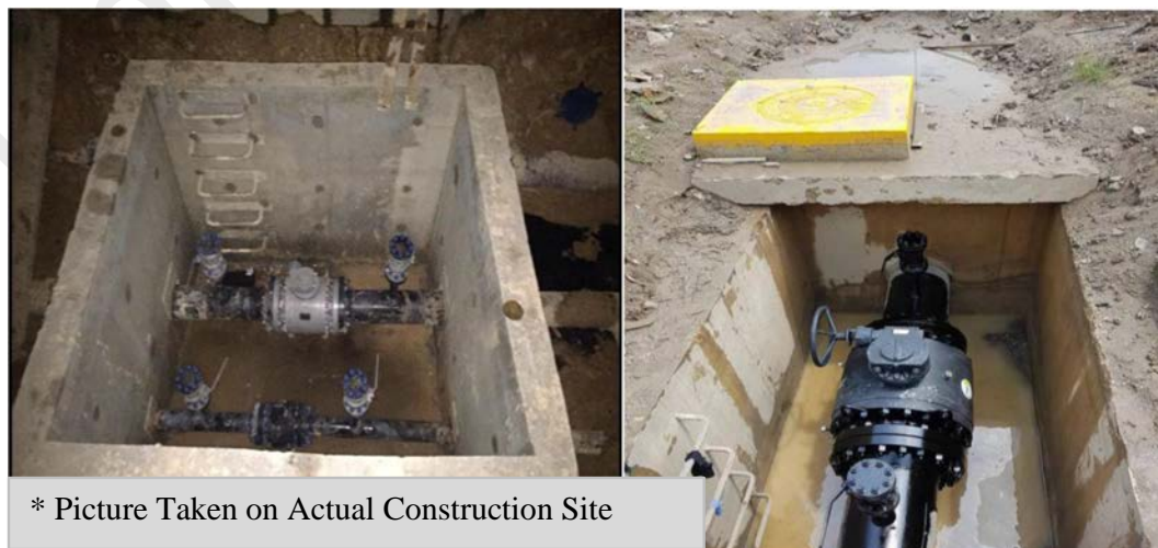
Figure 4.12: example of a valve chamber considered as a confined space.
