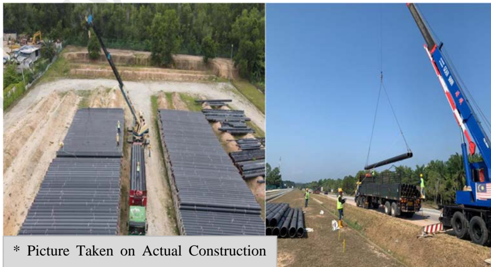
Figure 4.18: Pipe loading and unloading activities.
