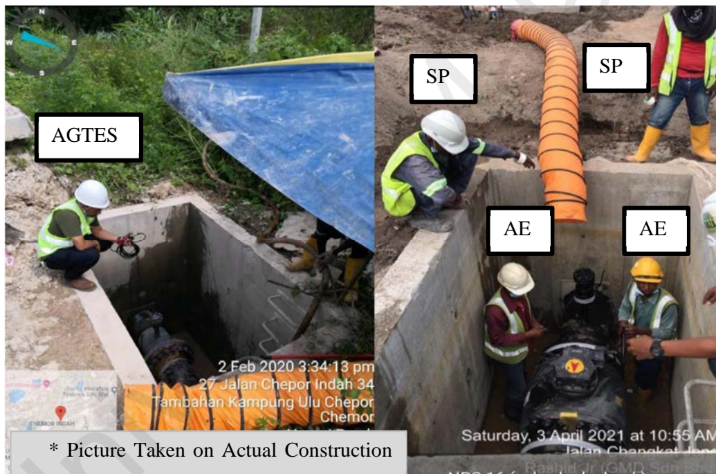
Figure 4.13: Safe confined space work practice.
