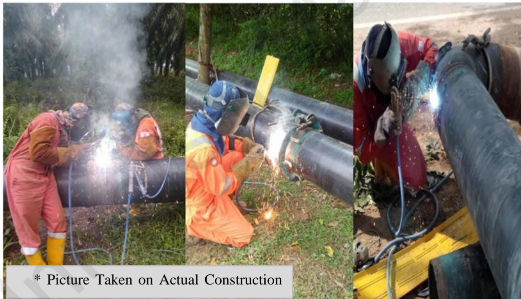
Figure 4.14: Pipeline welding activities.
