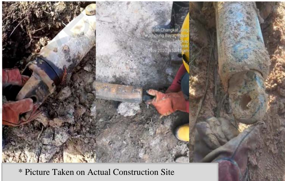
Figure 4.28: Testing swivel before attaching to rod for pipe pulling.
