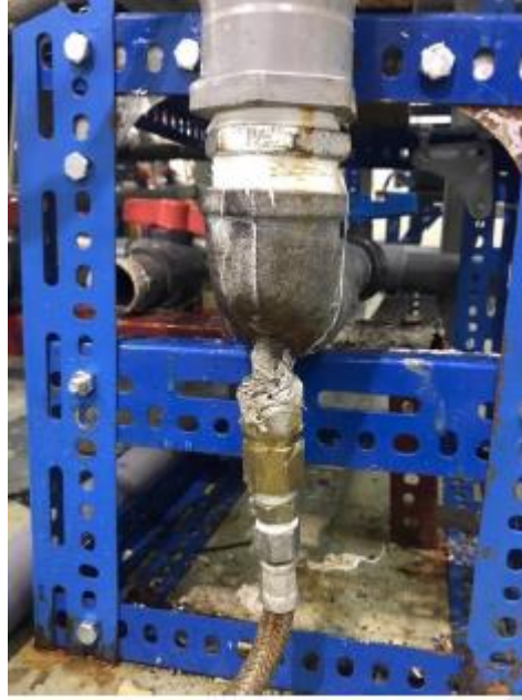
Figure 3.3: Welded Fitting to Inject Air.
