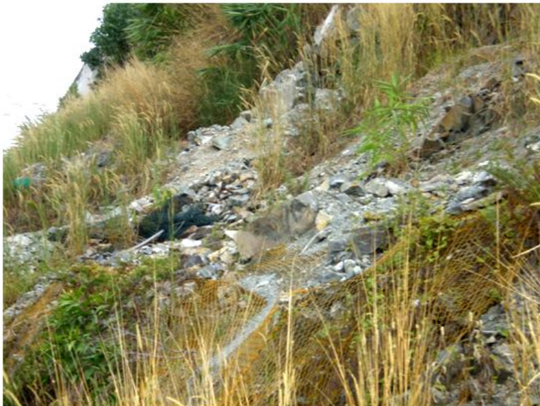
Fig. 5.3b. Hanging nets protecting the tumbling blocks at the base of the cut.
