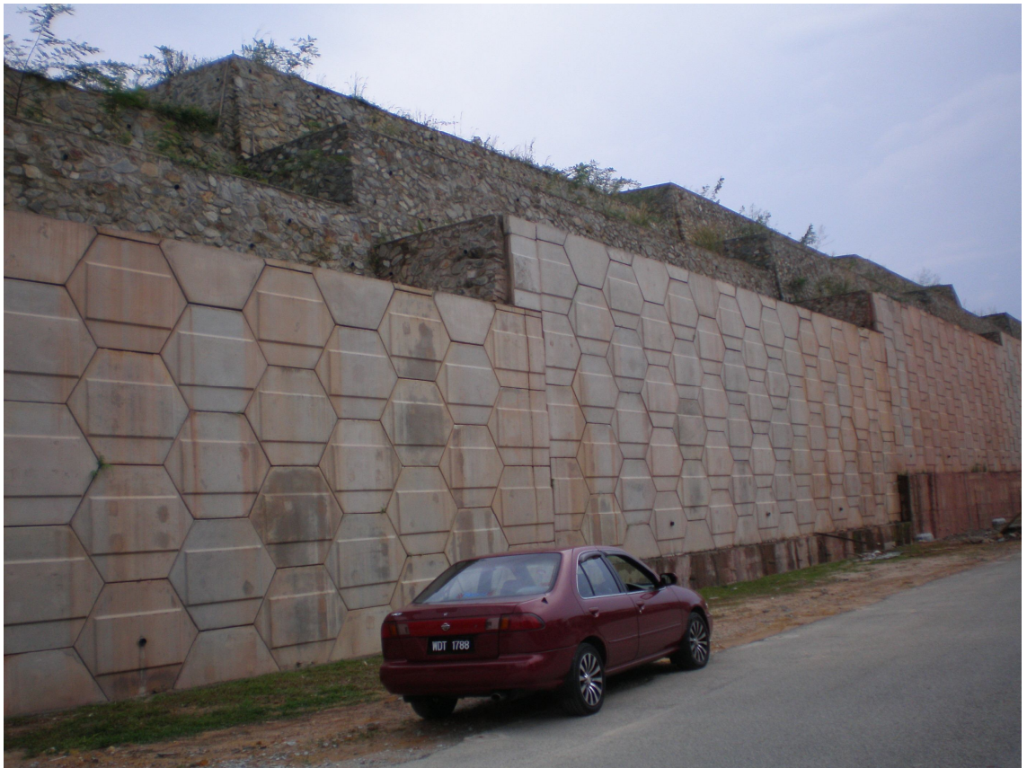
Fig. 5.9. Retaining walls in Taman Ukay Perdana.
