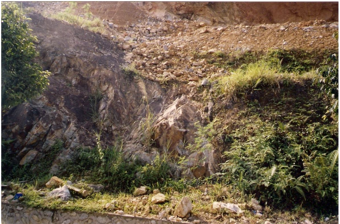
Fig.5.1. Shallow slips at older unbenched cuts.
