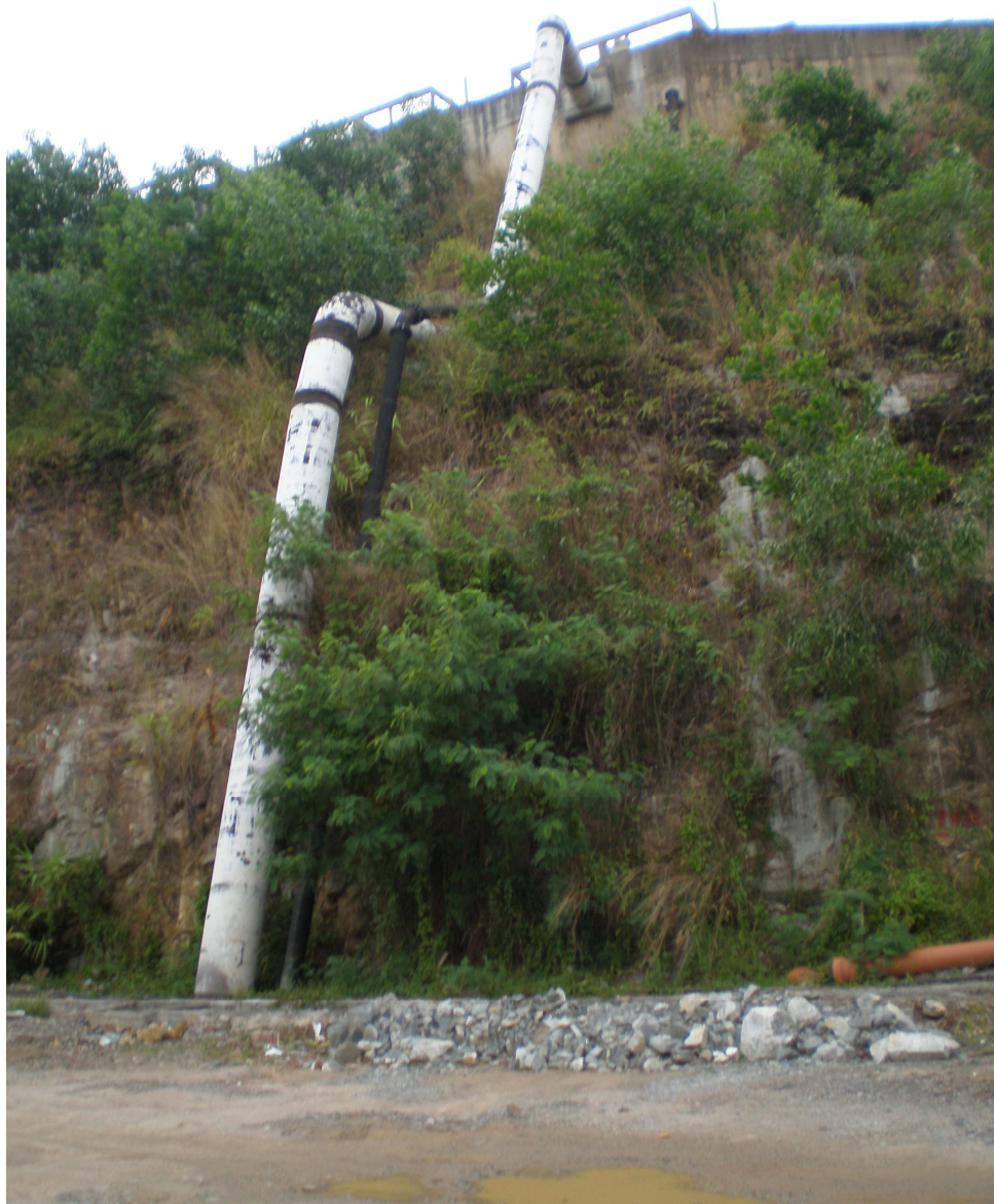
Fig. 5.10a. Drainage hose from Summer Set residential units down the slope.
