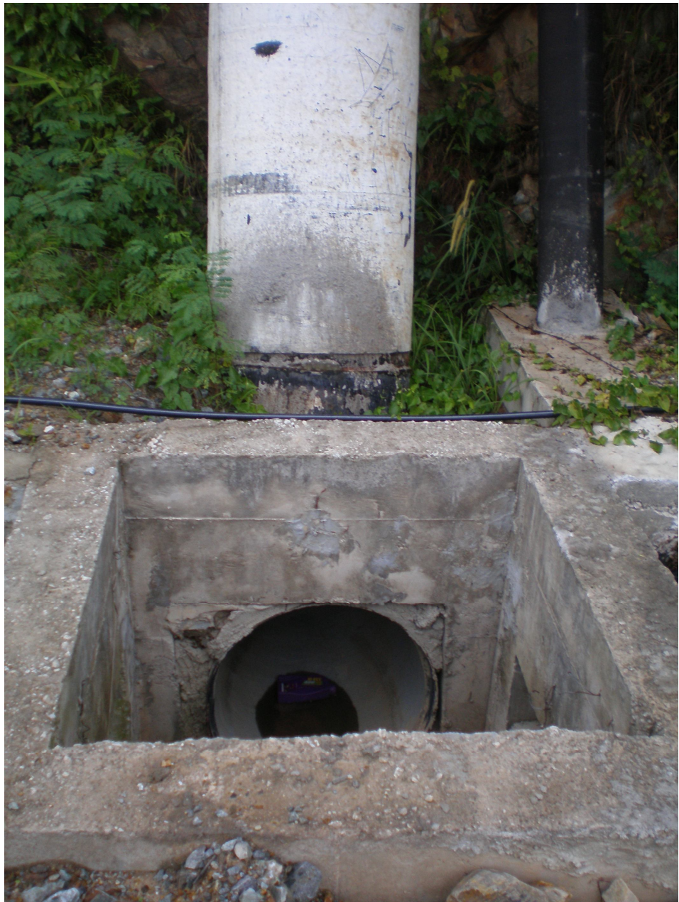
Fig. 5.10b. The drainage hose empties into the gutter drain at the foot of the slope.
