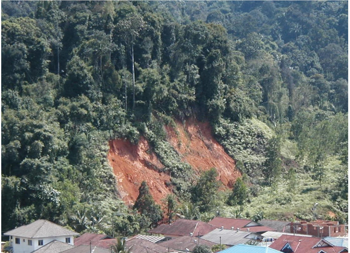
Fig. 5.6: A slump type of failure adjacent to Sri Baiduri apartment.
