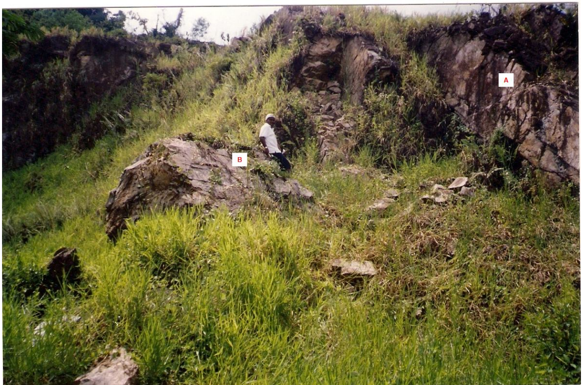
Fig.5.2. Topple in Jalan UP5/7. The rock block in position “B” overturned from position “A” due to cross jointing, the block weight, and stress relief forces.
