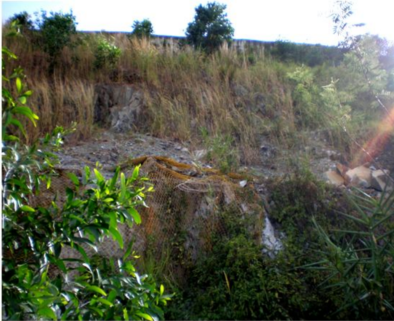
Fig. 5.3a. Photograph of the complex failure involving rockfalls and planar sliding
