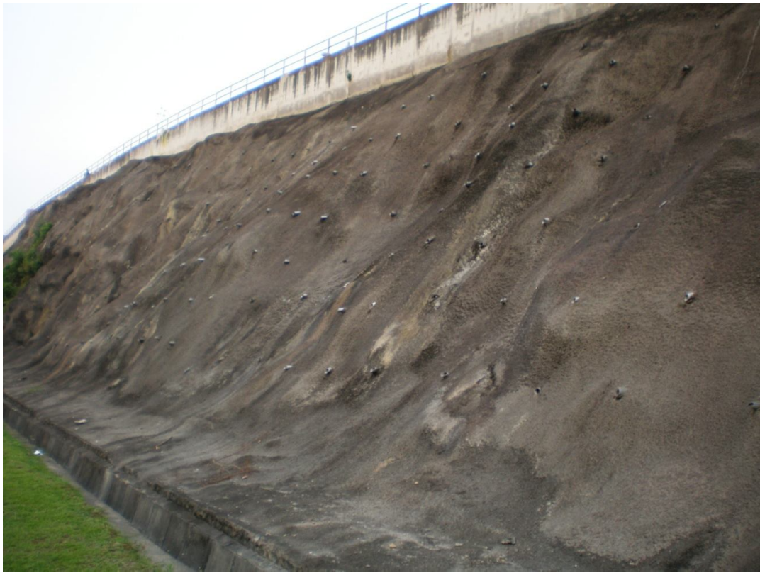
Fig.5.7: Guniting – Wire mesh used with pipes almost half buried within the sprayed concrete.
