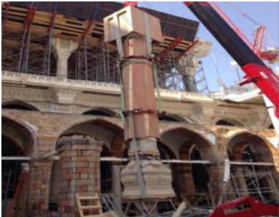
Figure 3.16: Column dismantling
