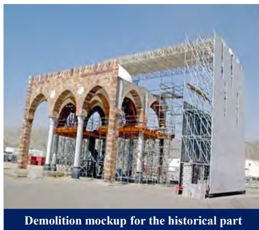
Figure 3.6: Demolition mockup for the historical and nonhistorical parts in the workshop area
