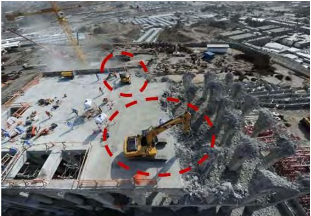
Figure 4.6: Large (in the bottom red circle) and small (in the top red circle) machinery at the demolition mockup
