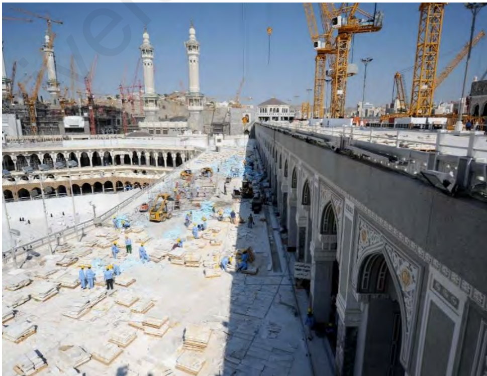
Figure 4.10: Marble and roofing system material removal
