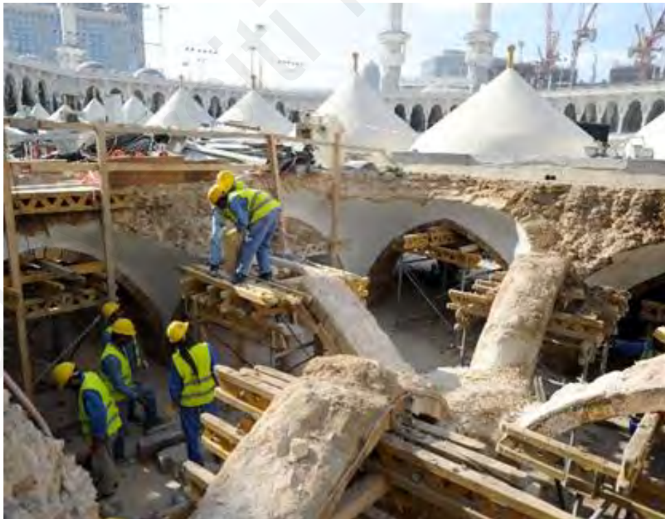
Figure 3.20: Arches stones dismantling
