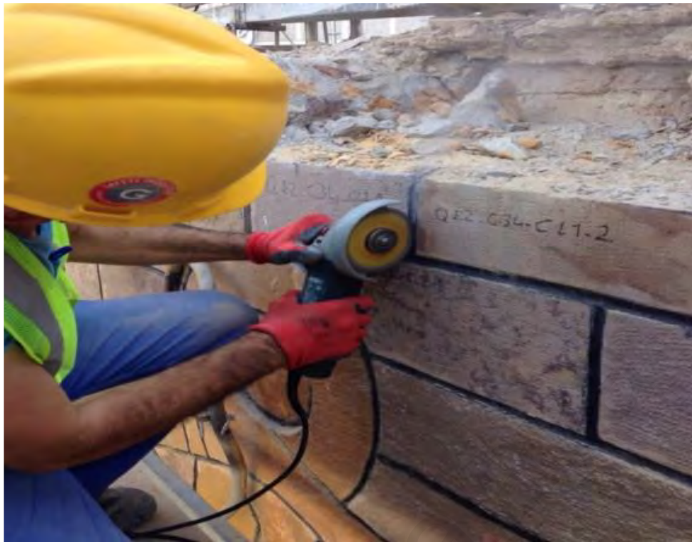
Figure 3.19: Facade stones dismantling
