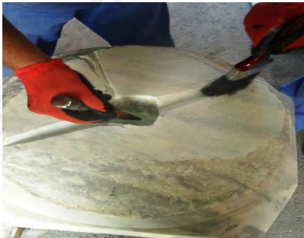
Figure 3.25: Surface cleaning of a column base
