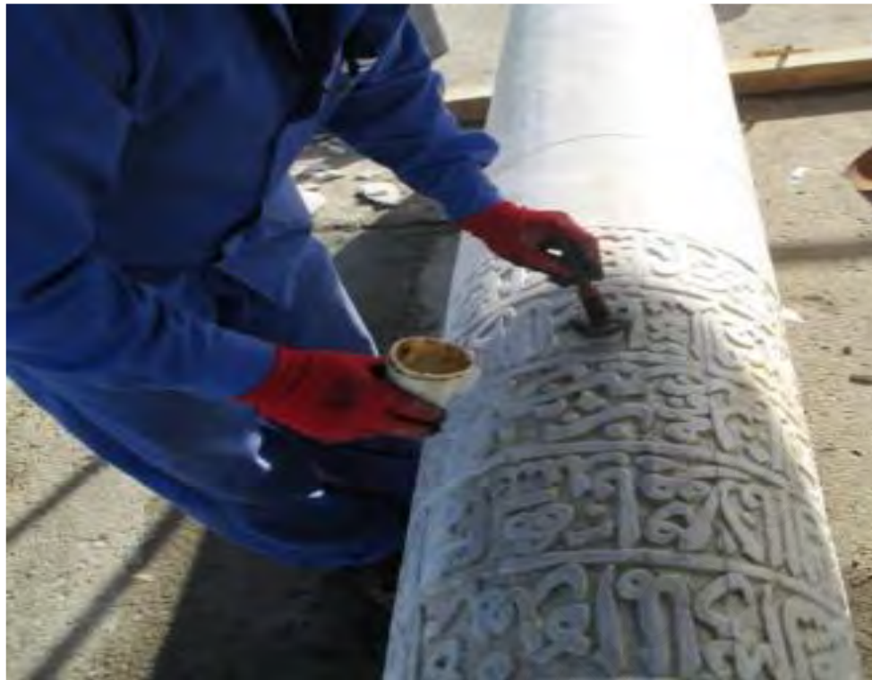
Figure 3.26: Deep cleaning of a column body
