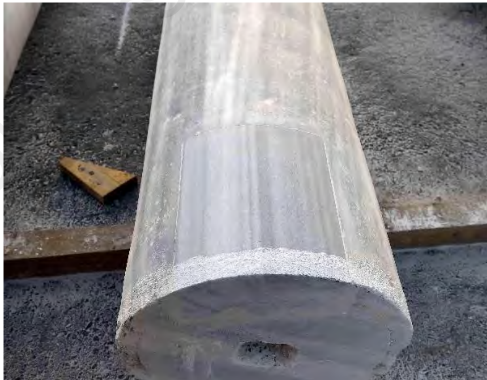
Figure 3.32: Marble column after restoration
