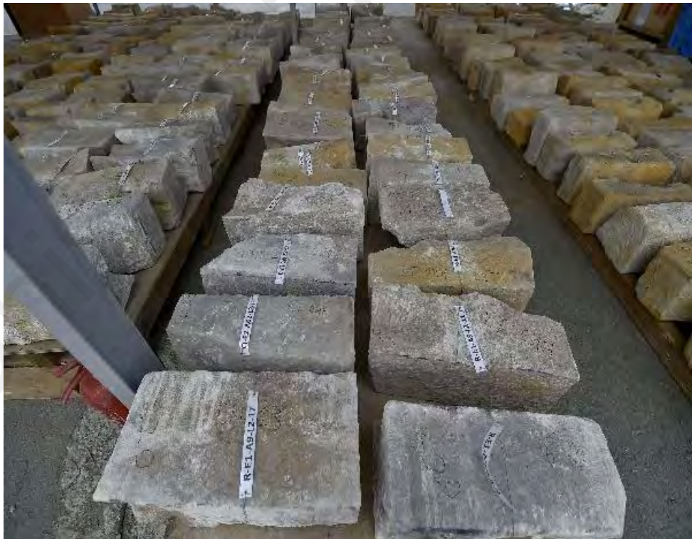
Figure 3.23: Sorting works of the stones
