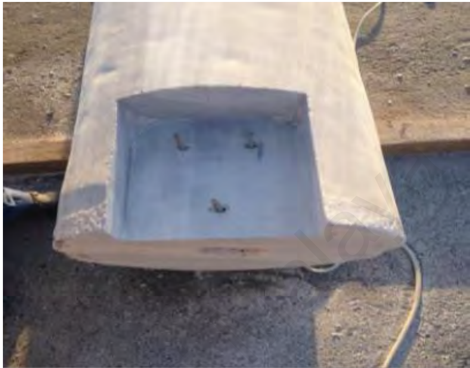
Figure 3.31: Chemical substances and anchors applied
