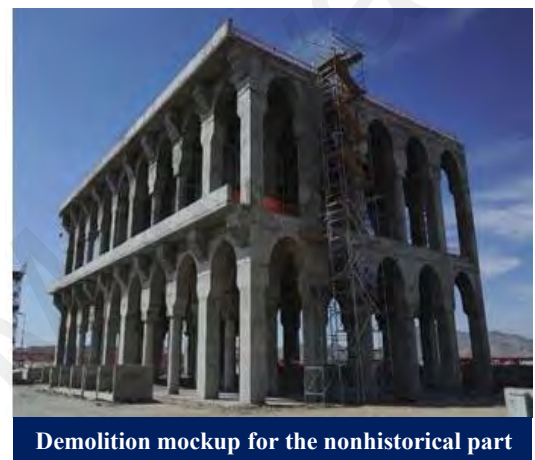
Figure 3.6: Demolition mockup for the historical and nonhistorical parts in the workshop area
