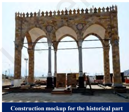
Figure 3.7: Construction mockup for the historical and nonhistorical parts in the workshop area
