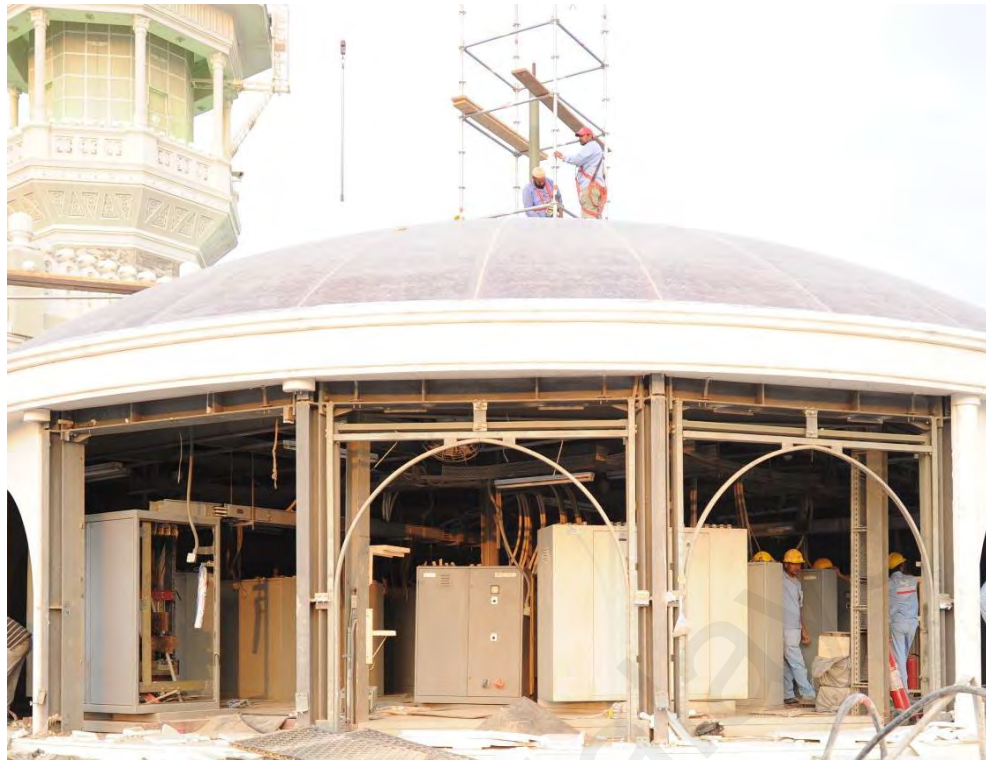
Figure 4.11: Rerouting work for an electrical service room
