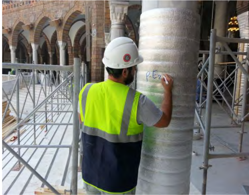
Figure 3.13: Numbering the column body
