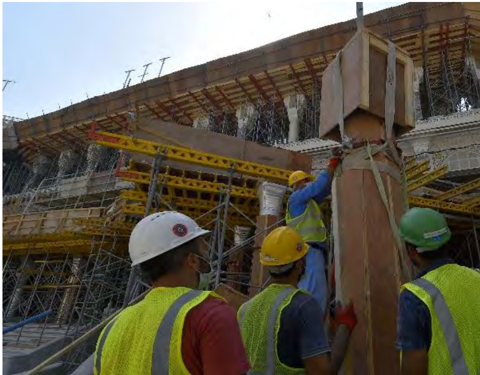
Figure 3.15: Protecting and packing the column
