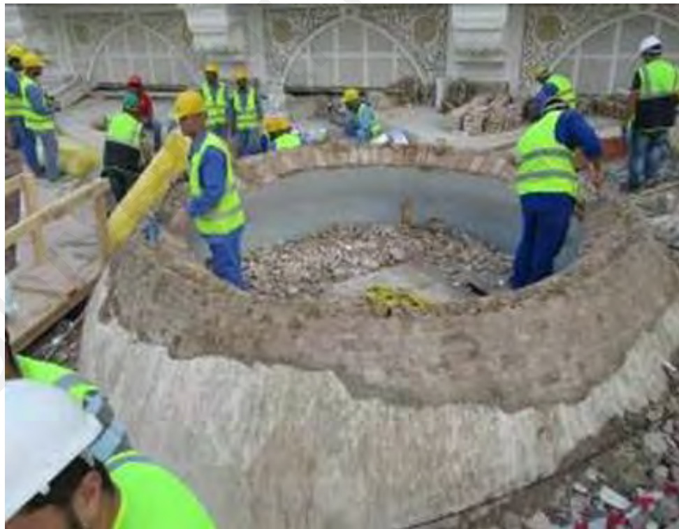
Figure 3.18: Domes dismantling
