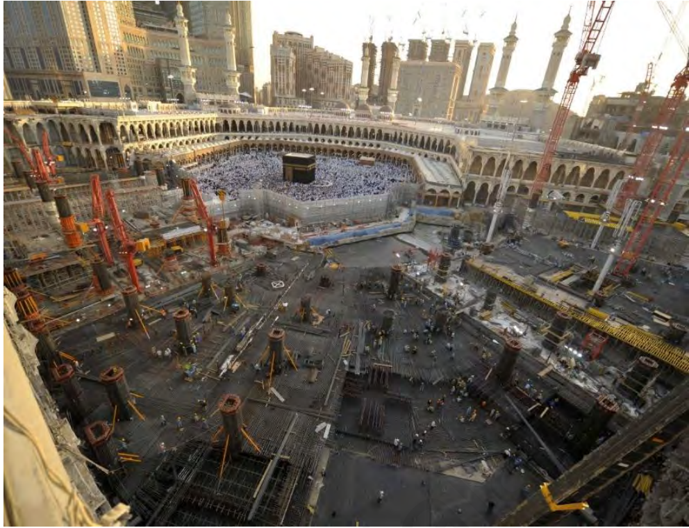
Figure 4.12: Steel reinforcement density in the raft foundation
