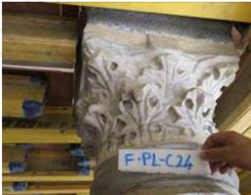
Figure 3.14: Numbering the column capital
