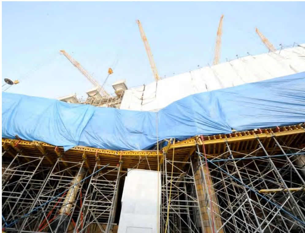
Figure 4.18: Back propping and supporting works
