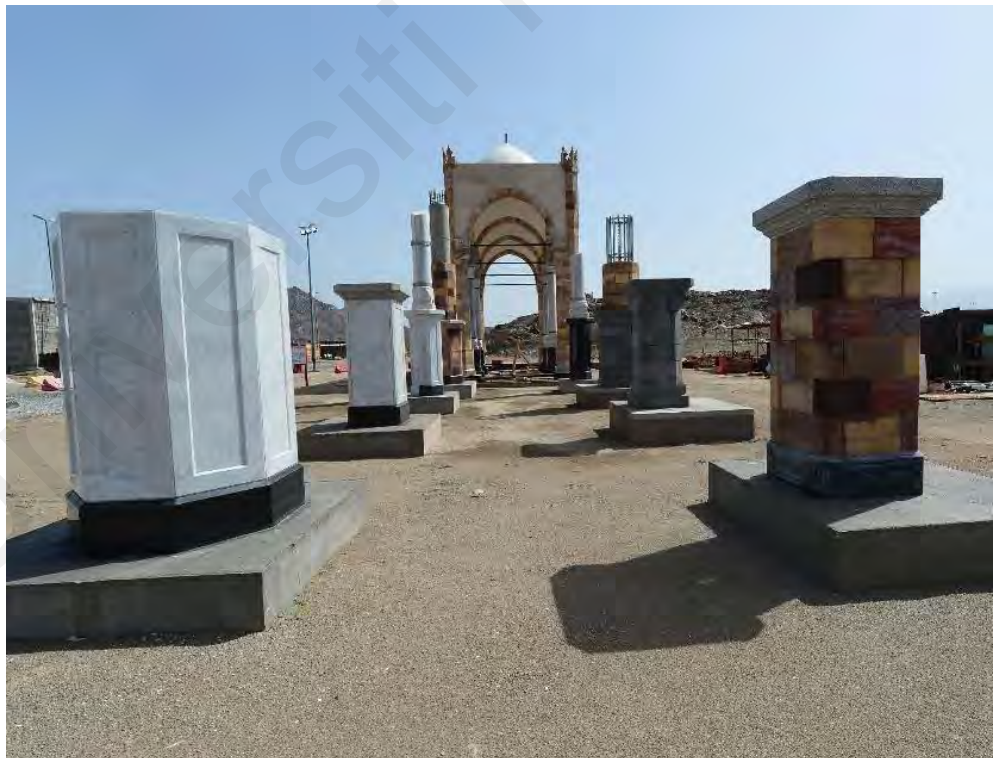
Figure 3.35: Mockups for column pedestals stone cladding
