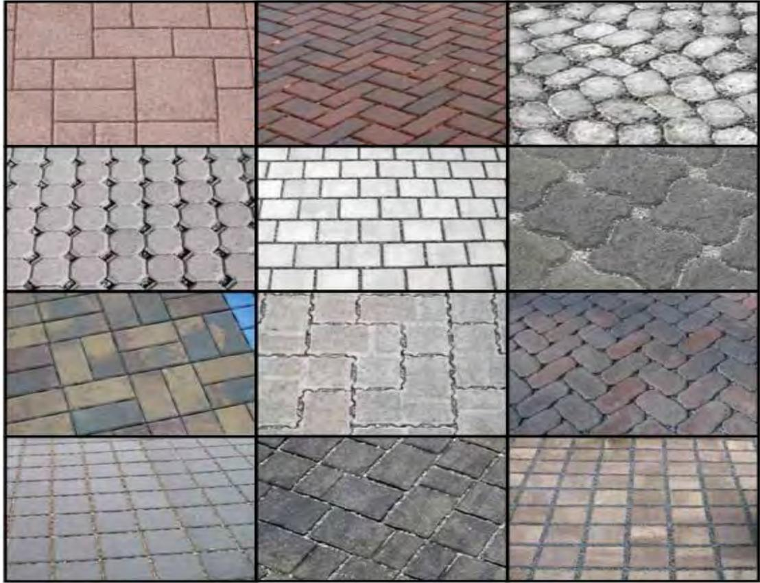
**Figure 2.4: Various types of PICP (Source: ICPI, 2013)**
