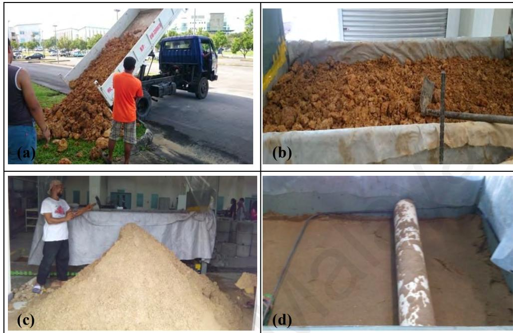
**Figure 3.16: Preparation of subgrade soils**
