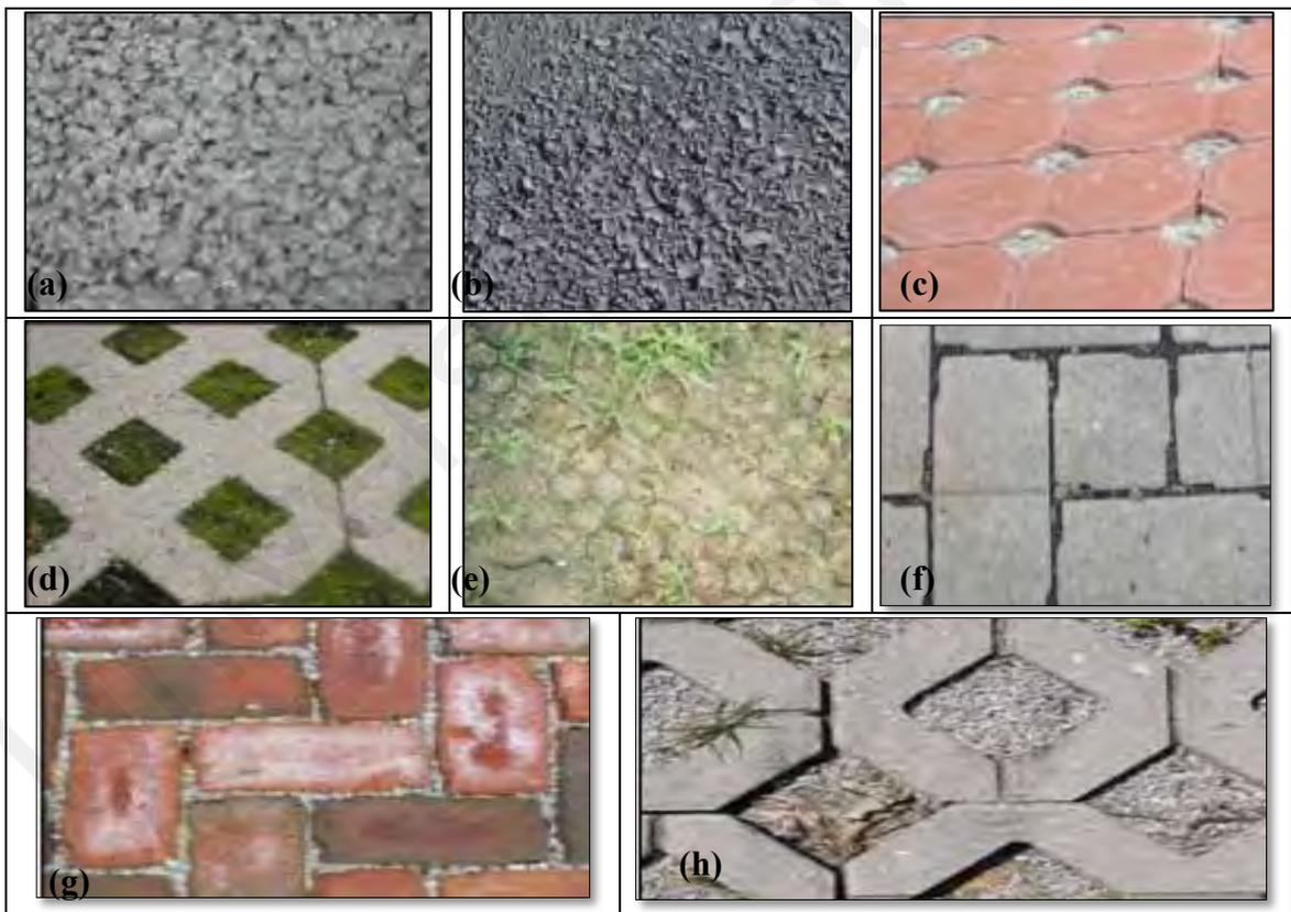
**Figure 2.3: Different types of permeable pavement (a) PC, (b) PA, (c) PICP with pea gravel fill, (d) PICP grid with topsoil and grass fill, (e) PICP plastic reinforcement with earth and grass fill (Source: Collins, 2007) and (f) PICP with concrete brick, (g) PICP with clay brick, and (h) PICP concrete grid with gravel fill (Source: Agouridis et al., 2011)**
