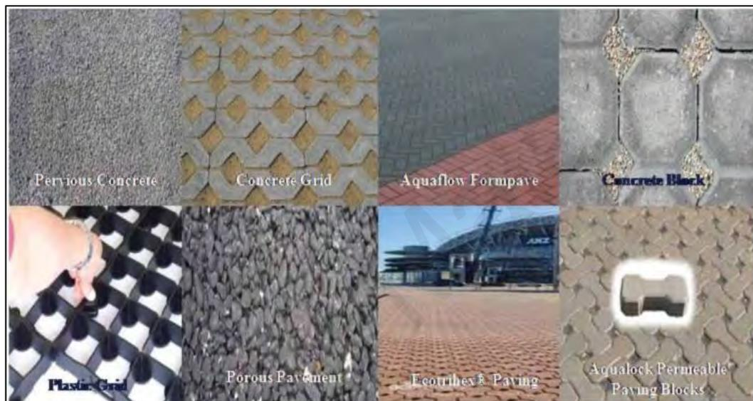
**Figure 2.5: Various types of PP system (Source: Imran et al., 2013)**
