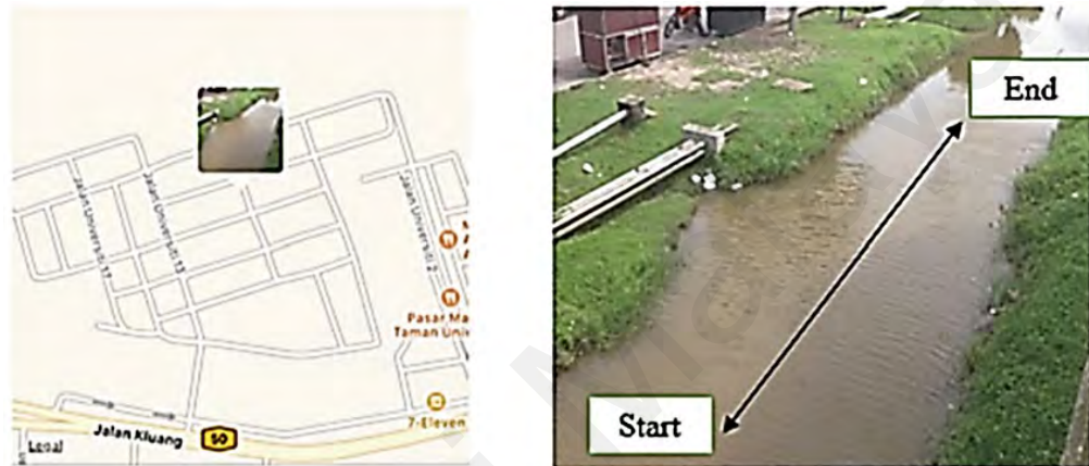
Figure 2.25: Navigating the trench near Taman University (Dahlan et al., 2019)
