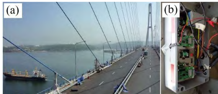
Figure 2.32: (a) Russky Bridge, Russia and (b) real-time decentralized controllers with PWM (Weber & Distl, 2015)
