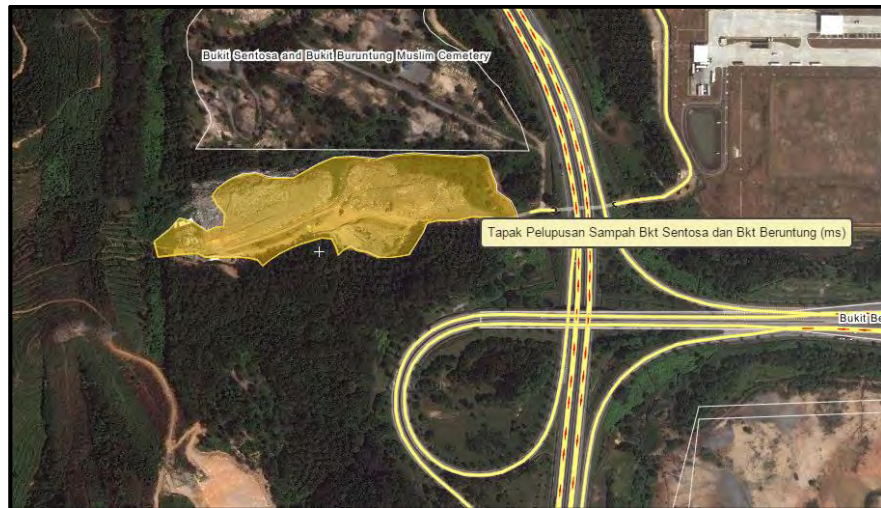
Figure 3.1: Bukit Beruntung disposal site ( https://goo.gl/maps/ahFccZrdet12 )
