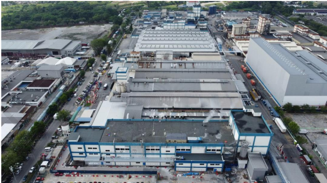
Figure 3.1: Birds Eye View of the Factory Complex
