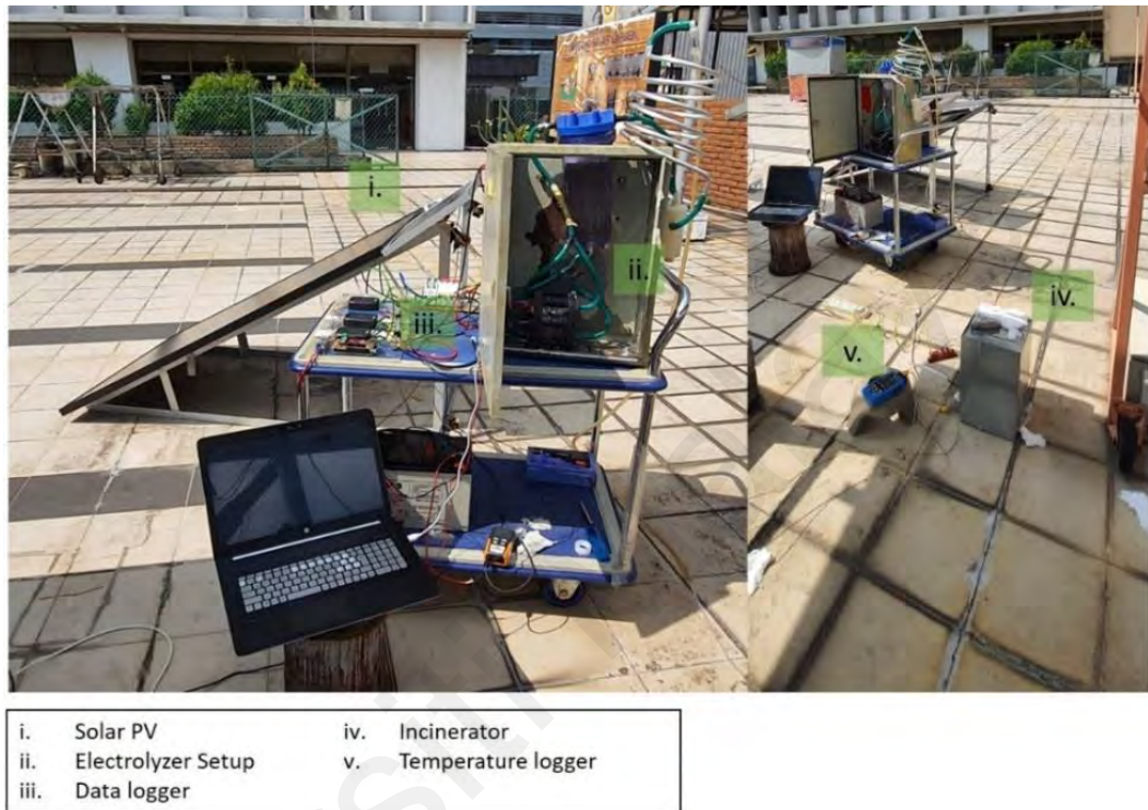
Figure 3.27 Outdoor setup for PV-ELE incineration
