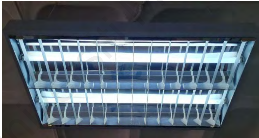
Figure 3.8: Fluorescent lamps installed in Wisma R&D (18 Watt)
