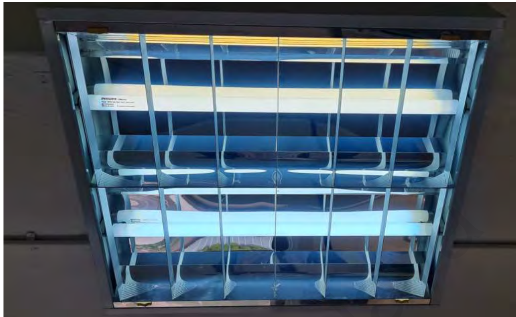
Figure 3.8: Fluorescent lamps installed in Wisma R&D (18 Watt)
