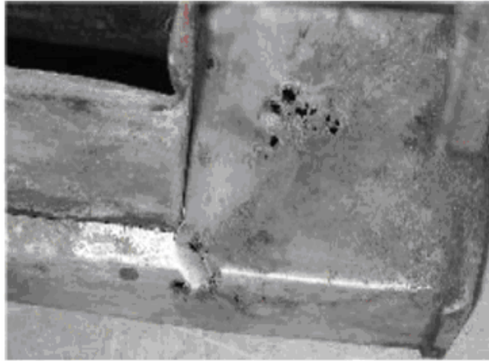
Figure 1.1 Show corrosion of steel (Kadry, 2008)
