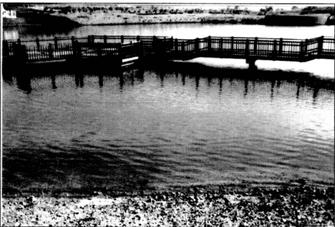
Figure 39. Water Sampling Point at PL10 after Construction of Wetland Cells
