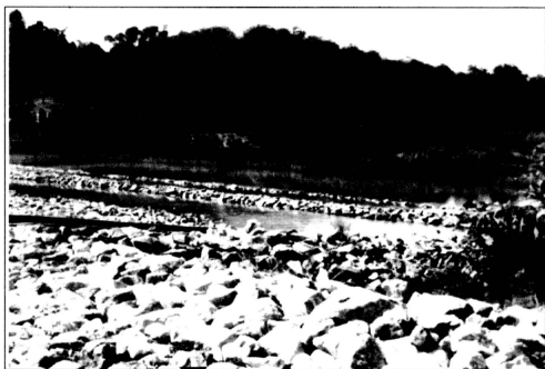
Figure 21. Water Sampling Point at UN5 after Construction of Wetland Cells
