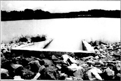
Figure 19. Water Sampling Point at UN7 after Construction of Wetland Cells
