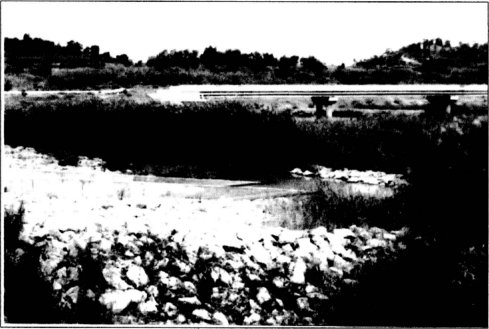
Figure 18. Water Sampling Point at UN8 after Construction of Wetland Cells
