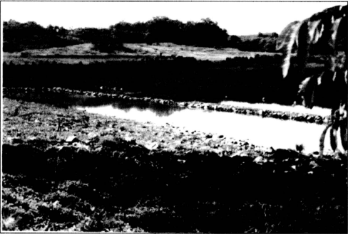
Figure 23. Water Sampling Point at UN3 after Construction of Wetland Cells
