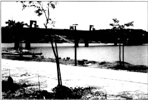
Figure 33. Water Sampling Point at PL4 after Construction of Wetland Cells
