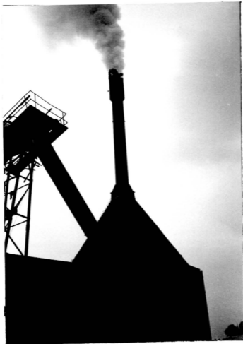
CORROSION OF INCINERATOR STACK
