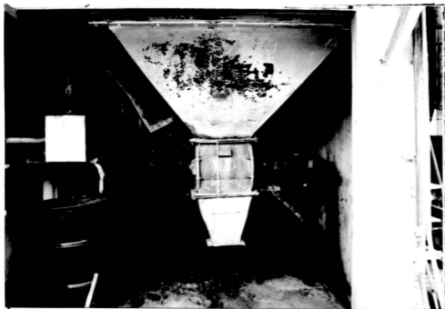
CORROSION OF MULTICLONE AND ROTARY AIR LOCK
