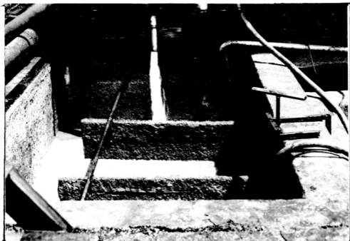
CONCRETE CORROSION IN EFFLUENT SUMP
