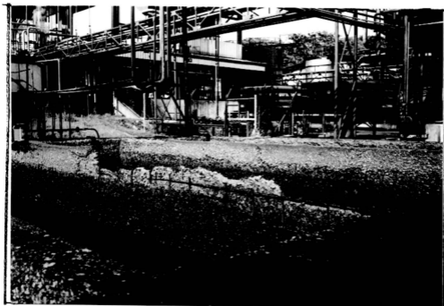
CONCRETE CORROSION IN RECIRCULATION BASIN
