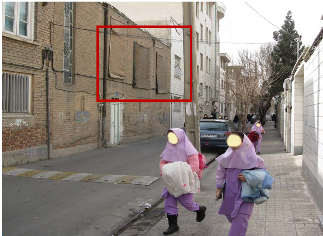
Figure 6. 1: the first floor windows are covered with curtains
