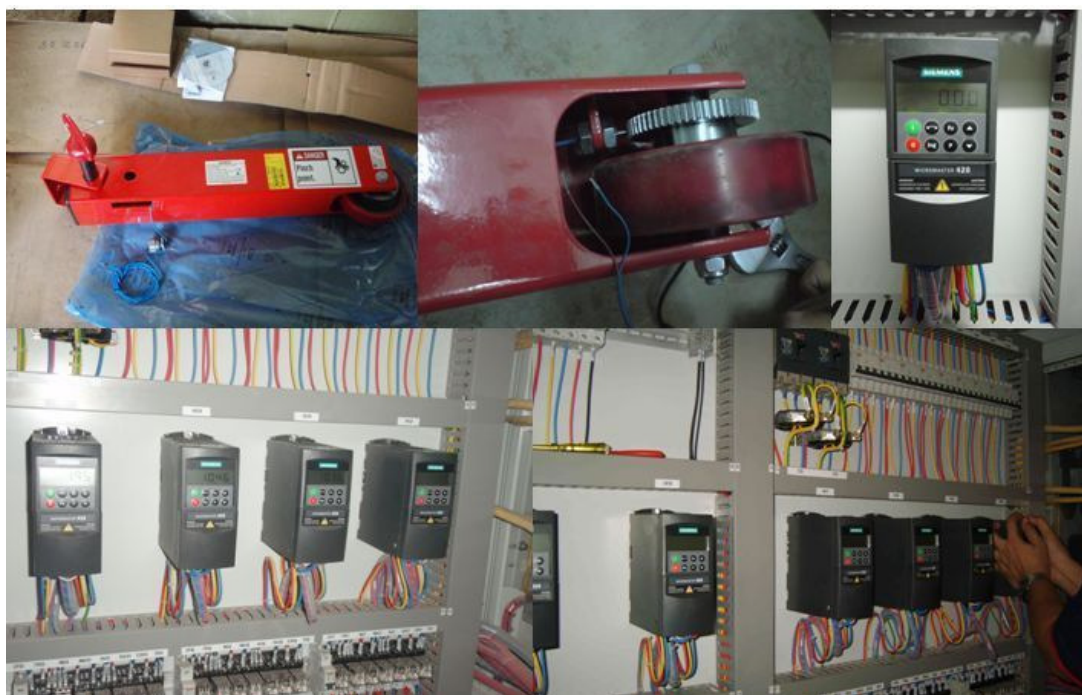
Figure 4.6 Installing PID on totalize weighing machine and how the PIDs are arranged
