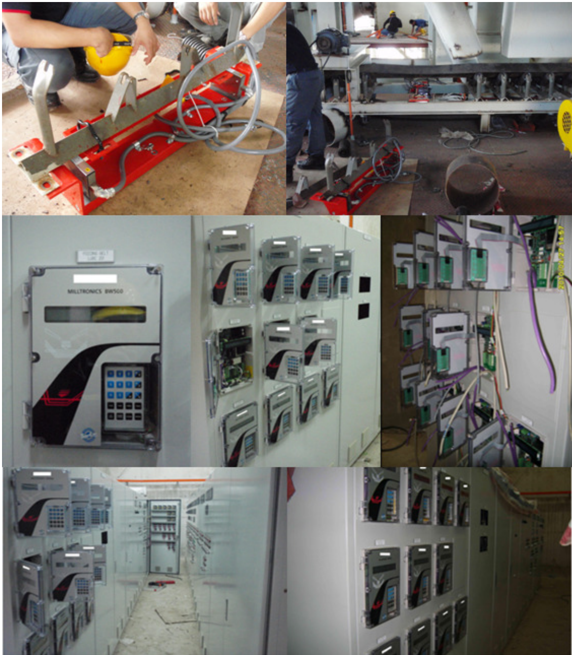
Figure 4.4 Installing PID on weight feeder and how the PIDs are arranged in a rack
