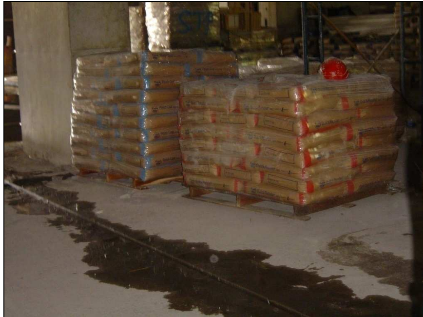
Figure 4.8: Storage of cement bags
