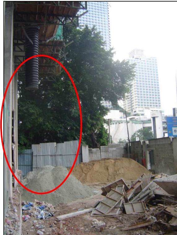
Figure 4.27: Rubbish chute attach to open space (dump area)
