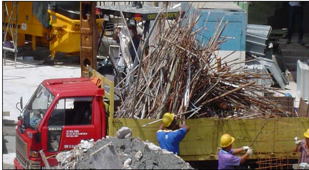
Figure 4.20: Steel waste ready to sent back to vendor for recycling
