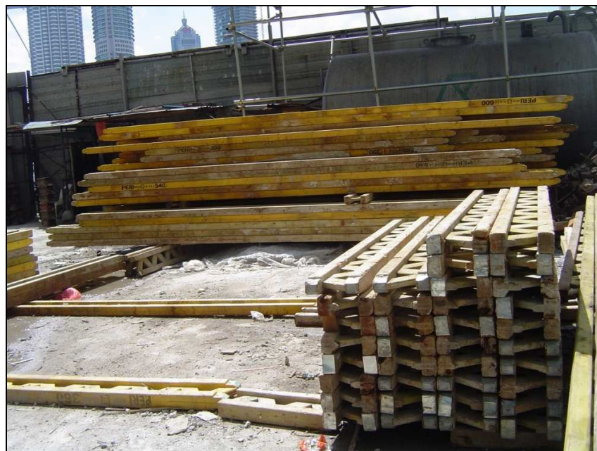
Figure 4.7: Storage of PERI formwork at open space
