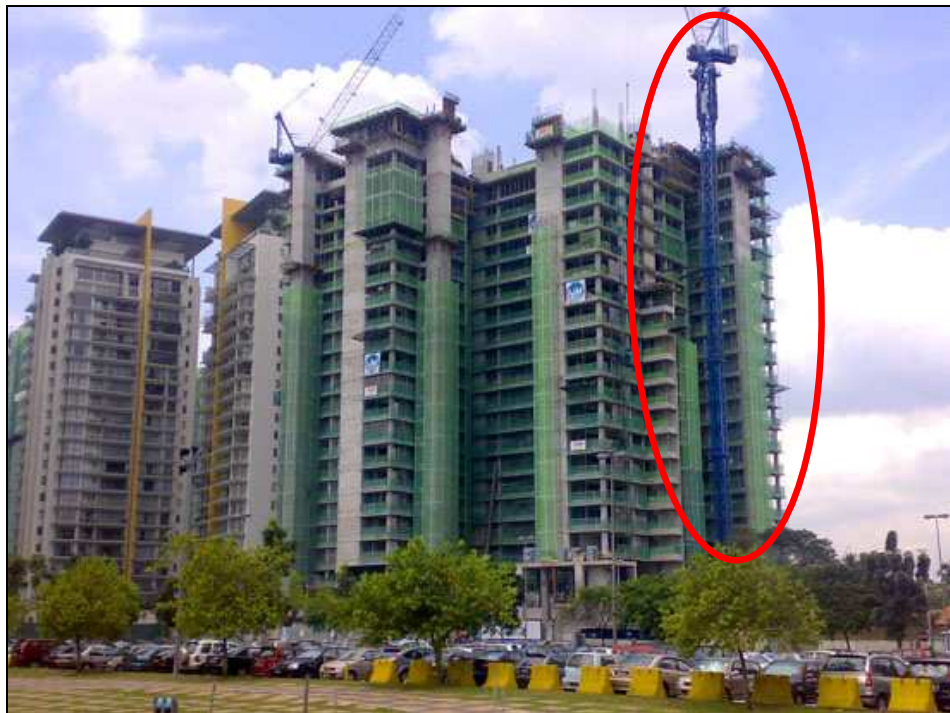
Figure 4.22: Tower crane
