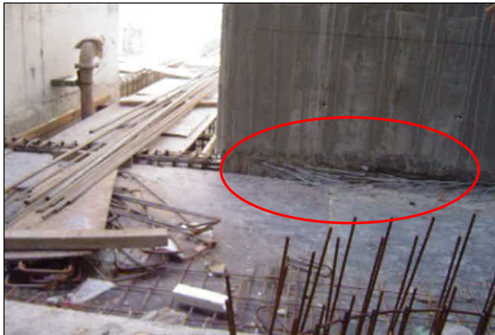
Figure 4.24: Hacking off concrete becomes waste
