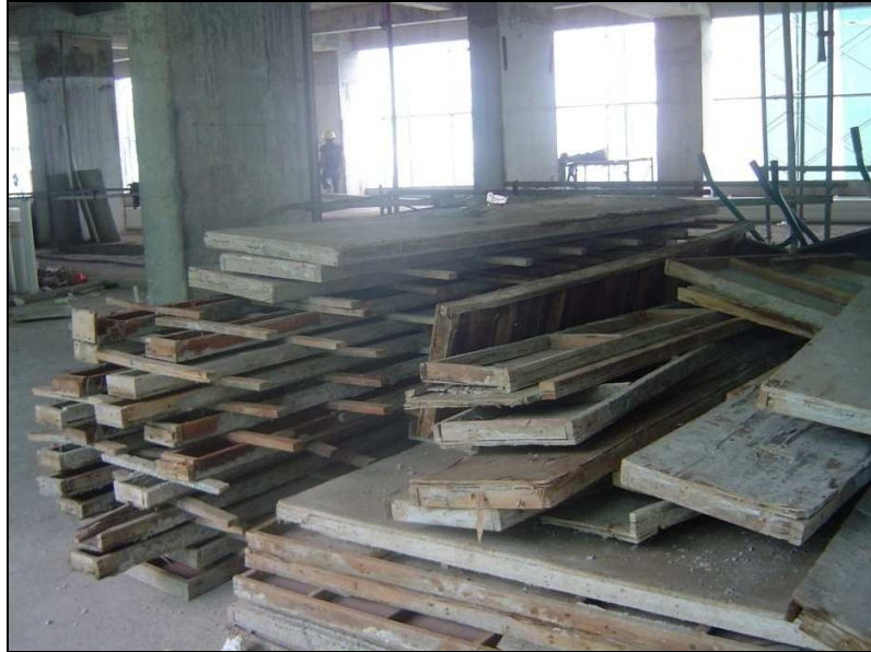
Figure 4.12: Storage of wood to be reused
