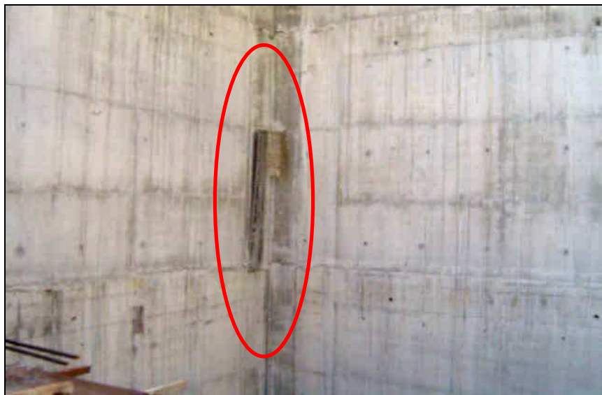
Figure 4.19: Jump system can cause wood waste (improper handling)
