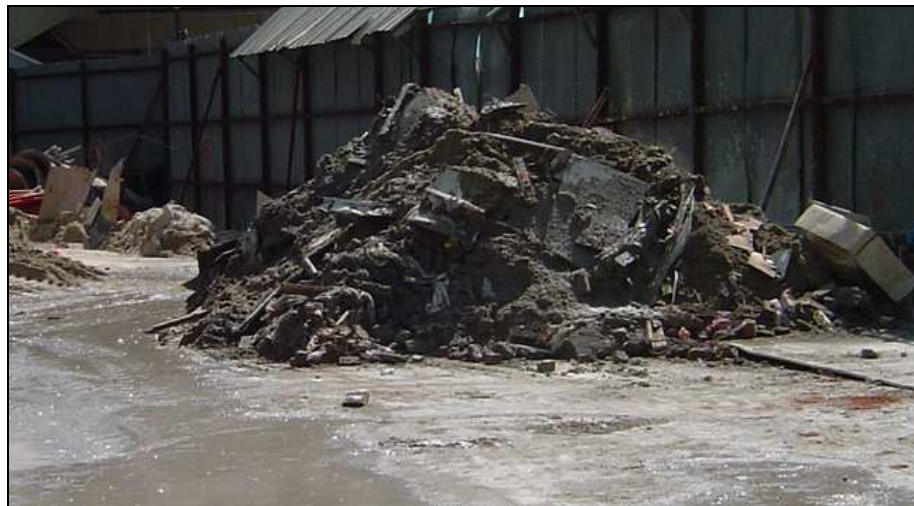
Figure 4.15: Waste materials are not segregated from useful material
