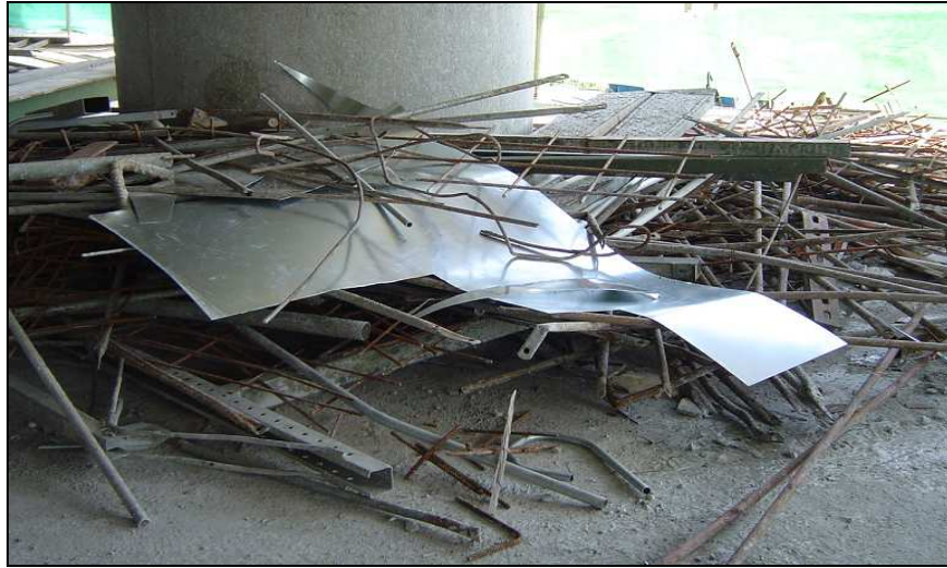
Figure 4.16: Cutting waste of reinforcement
