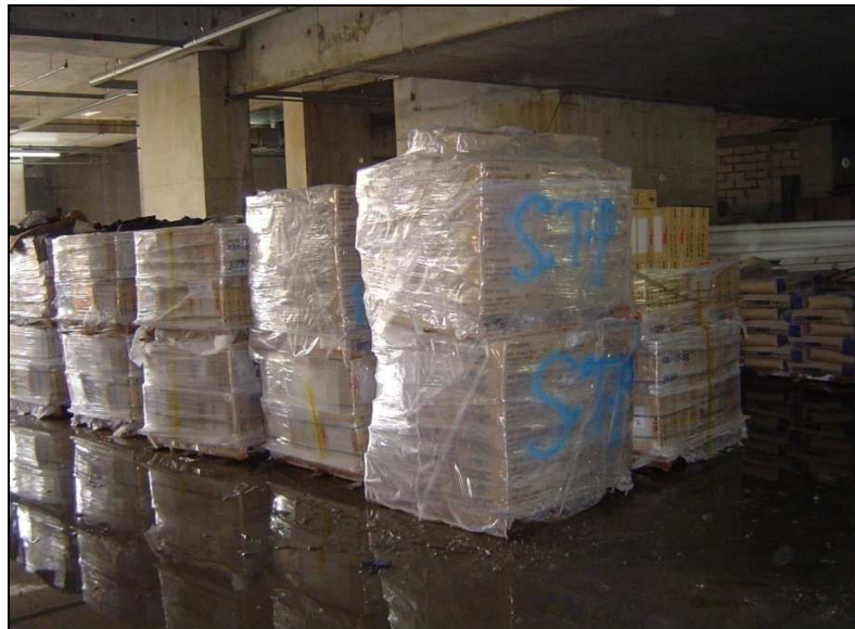
Figure 4.9: Storage of tiles at secured and under cover area (keep in original packaging until used)
