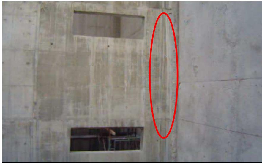
Figure 4.18: Incorrect dimension cause formwork giveaway
