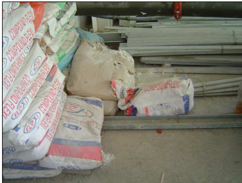
Figure 4.11: Improper storage of plaster
