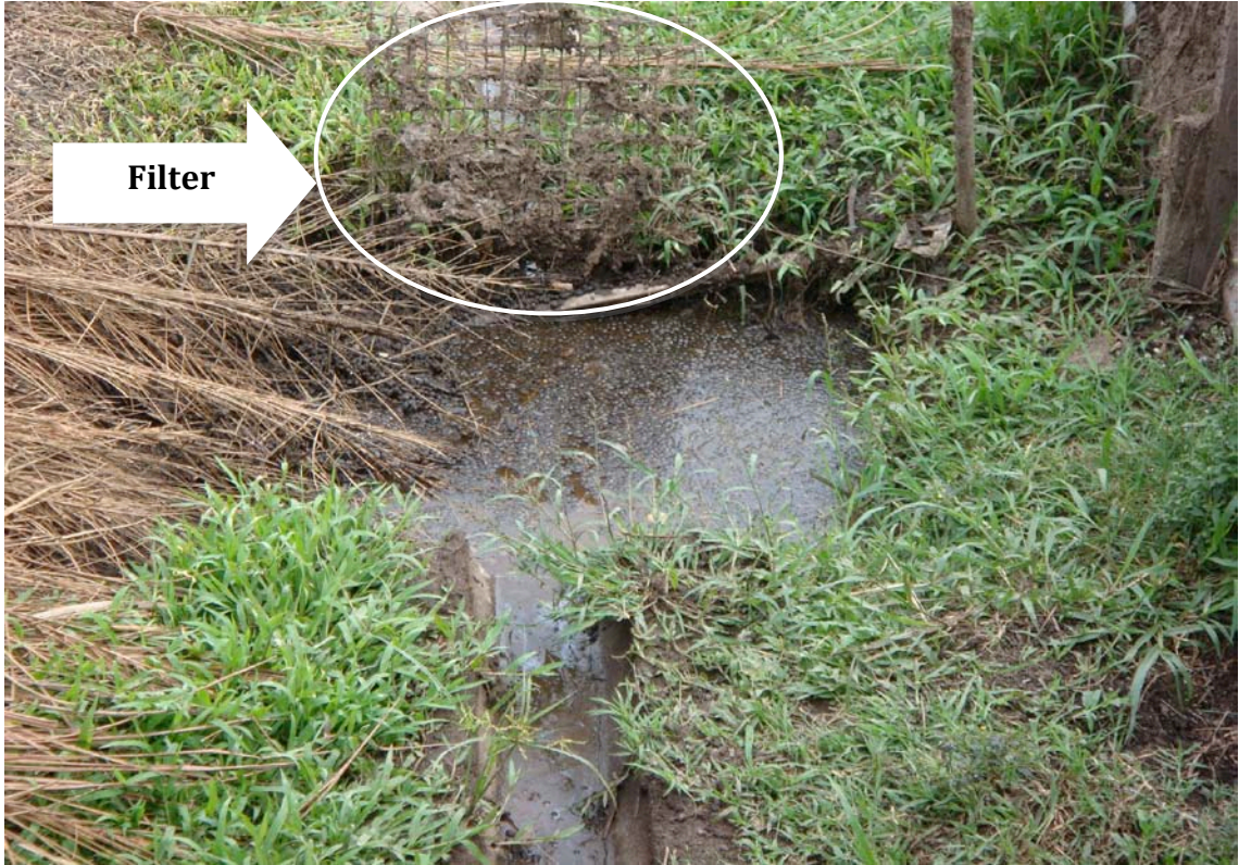
Figure 4.9 : Feces are separated by the filter before the wastewater enters the pond.
