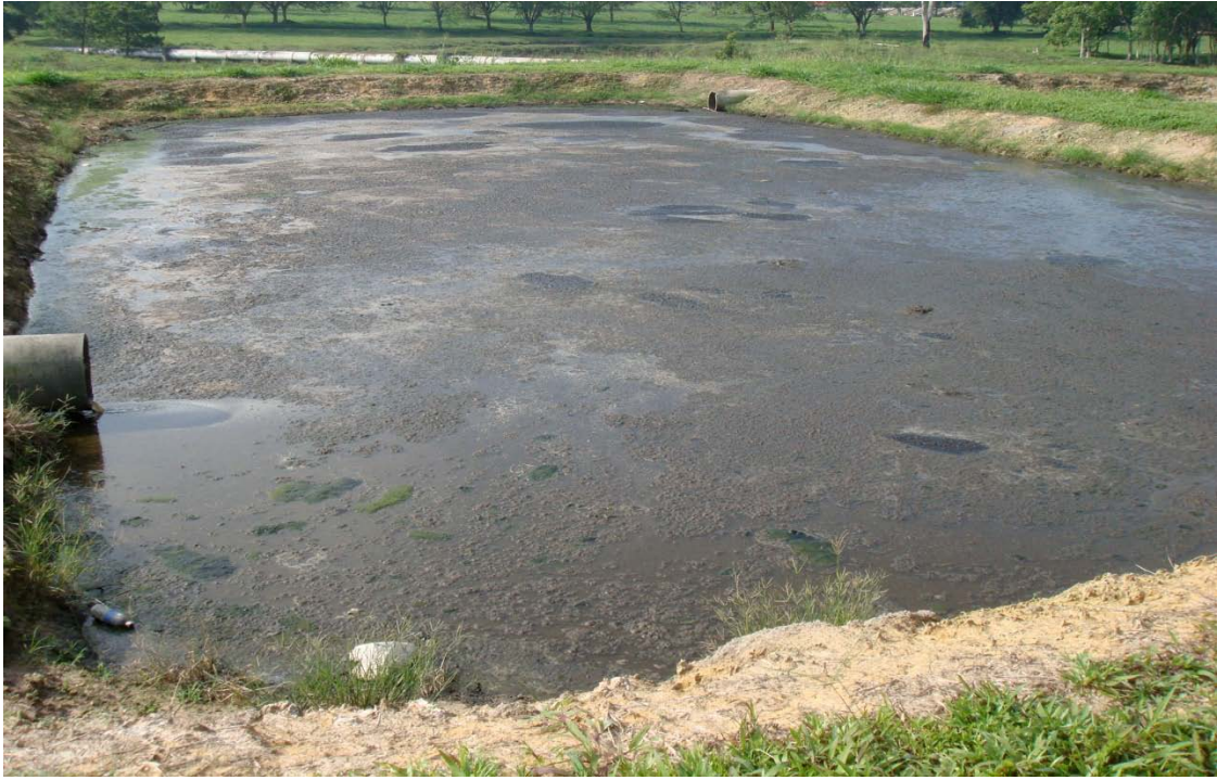
Figure 6.8 : Wastewater in the first pond undergone for sedimentation process.
