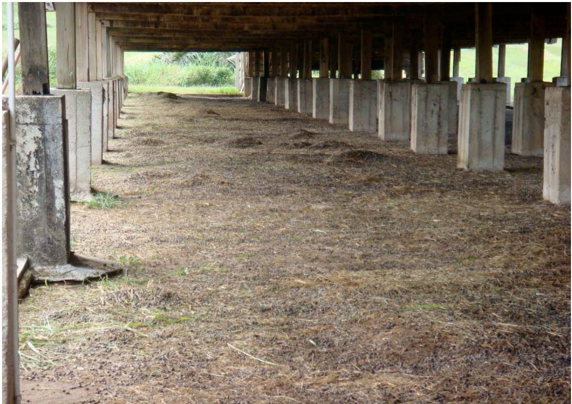
Figure 4.17 : Soil-based under the feedlot house at Farm D.
