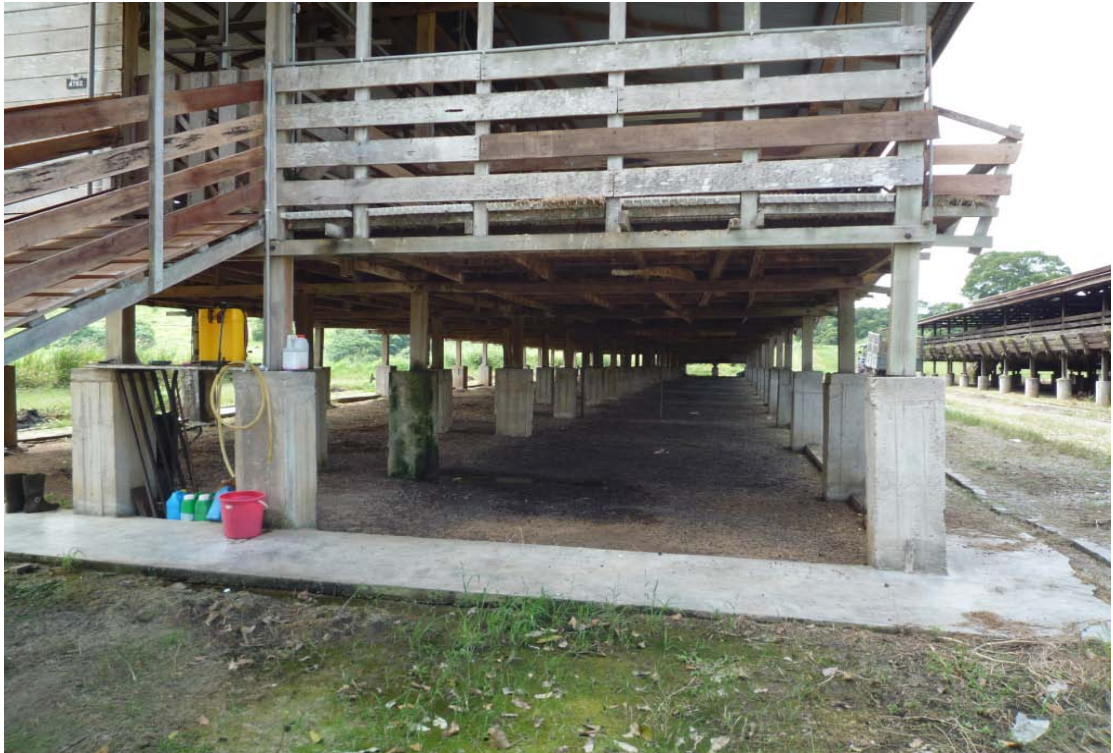
Figure 4.18 : Soil-based surrounded by cement concrete border at Farm D.
