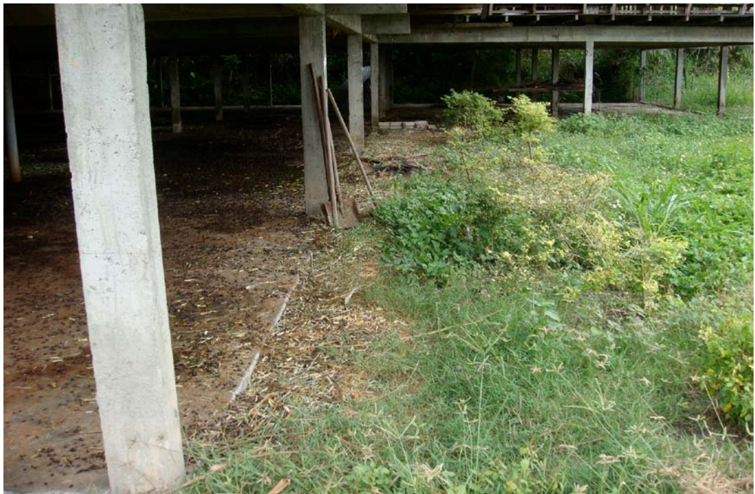
Figure 4.5 : Improper drainage system without end-point in feedlot area at Farm A.
