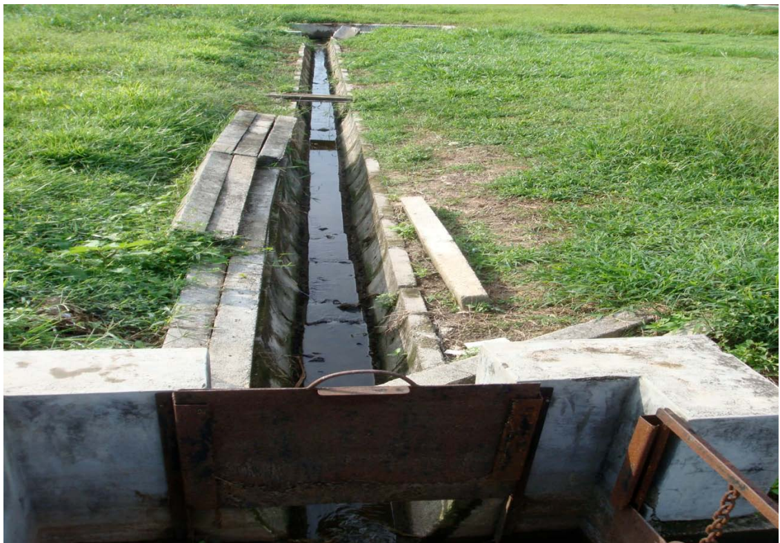
Figure 6.5 : Drainage that leads to treatment ponds from the separator tank.
