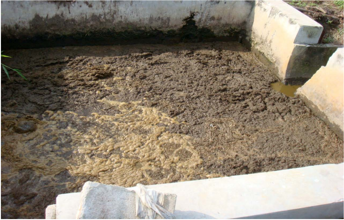
Figure 6.6 : Wastewater in holding pond before entering the inlet for treatment process.
