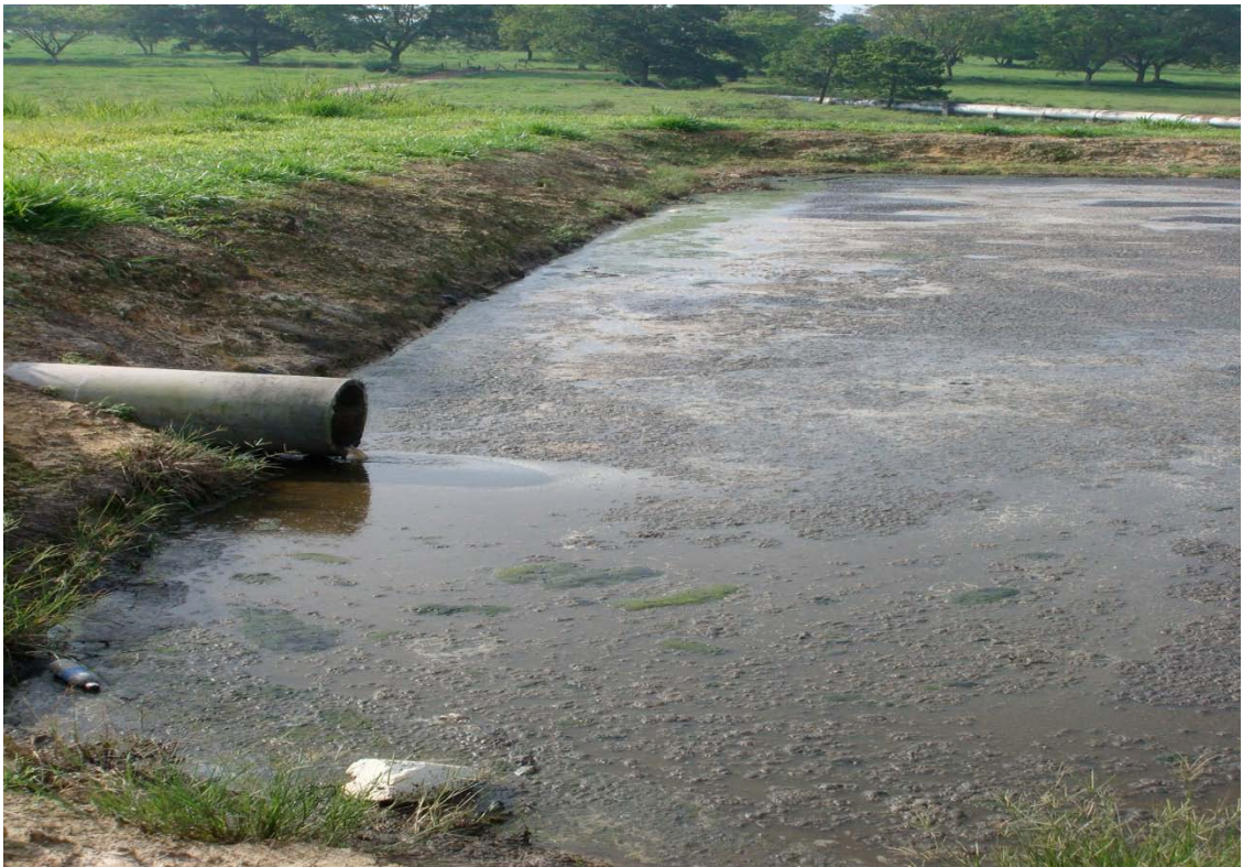
Figure 6.7 : Wastewater flowing from the holding pond through the concrete pipe.
