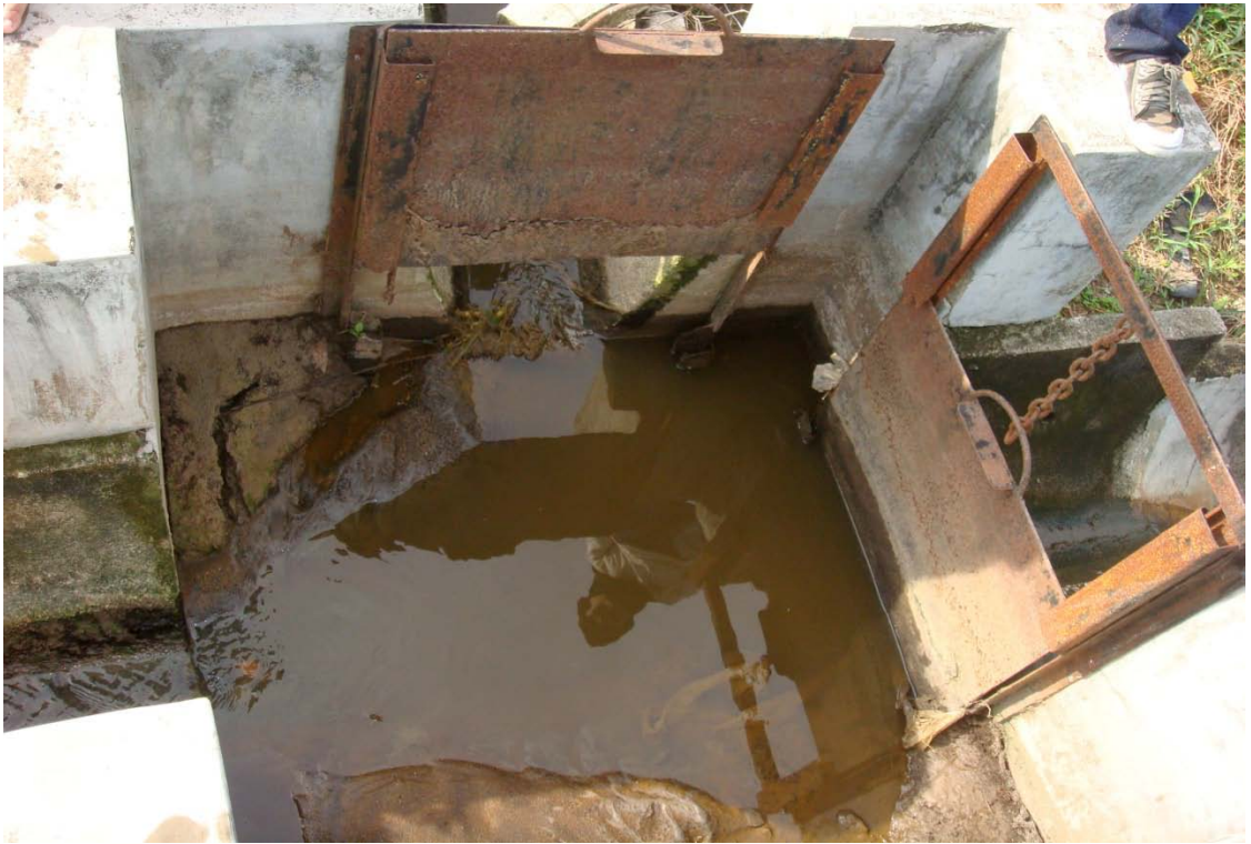
Figure 6.4 : Separator tank that separate the wastewater for release or treatment pond.
