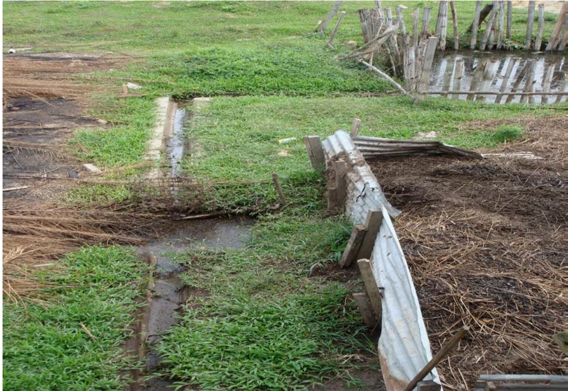
Figure 4.8 : A proper drainage system that flows the wastewater into a retention pond.
