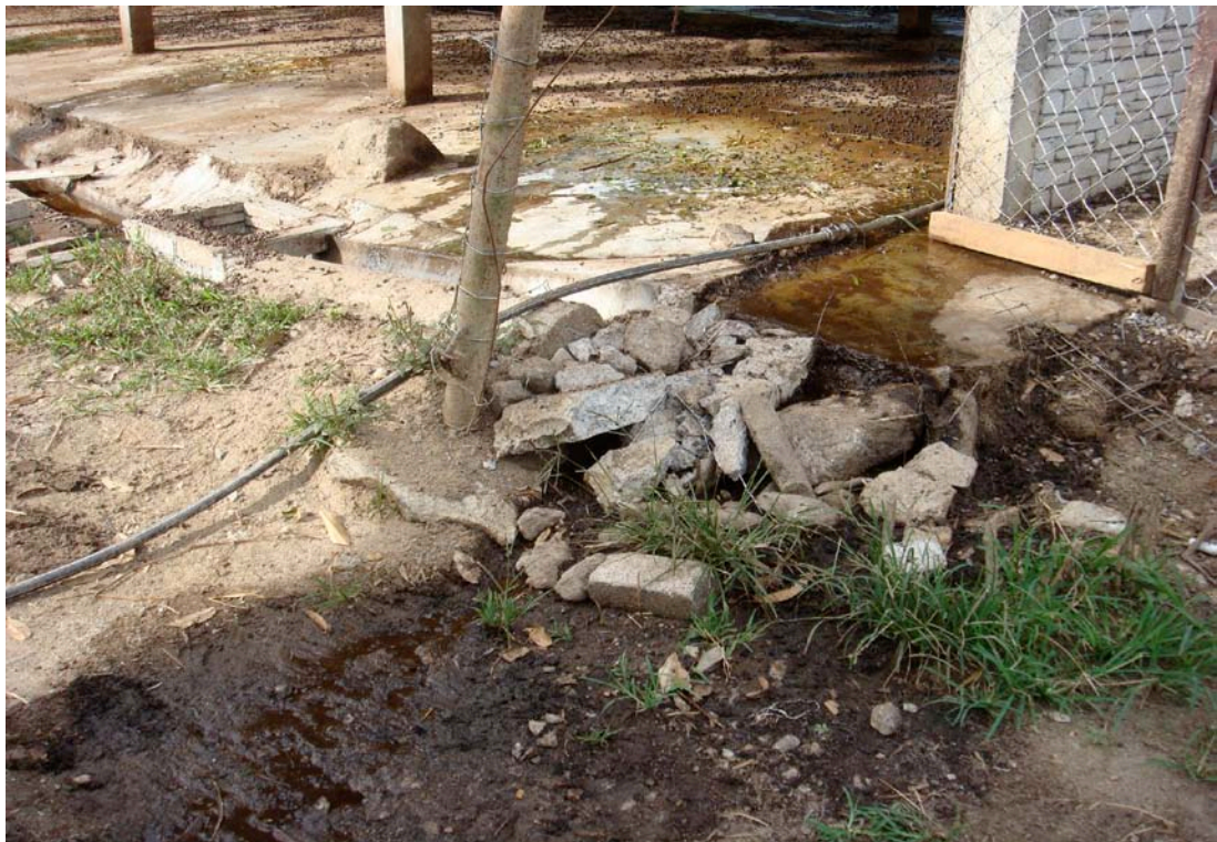
Figure 4.12 : Wastewater runoff caused by improper drainage system in Farm C
