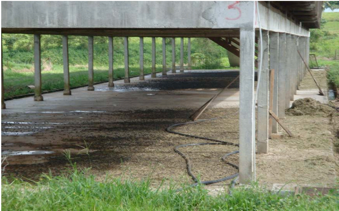
Figure 4.20 : A concrete-base at the feedlot area on Farm E.
