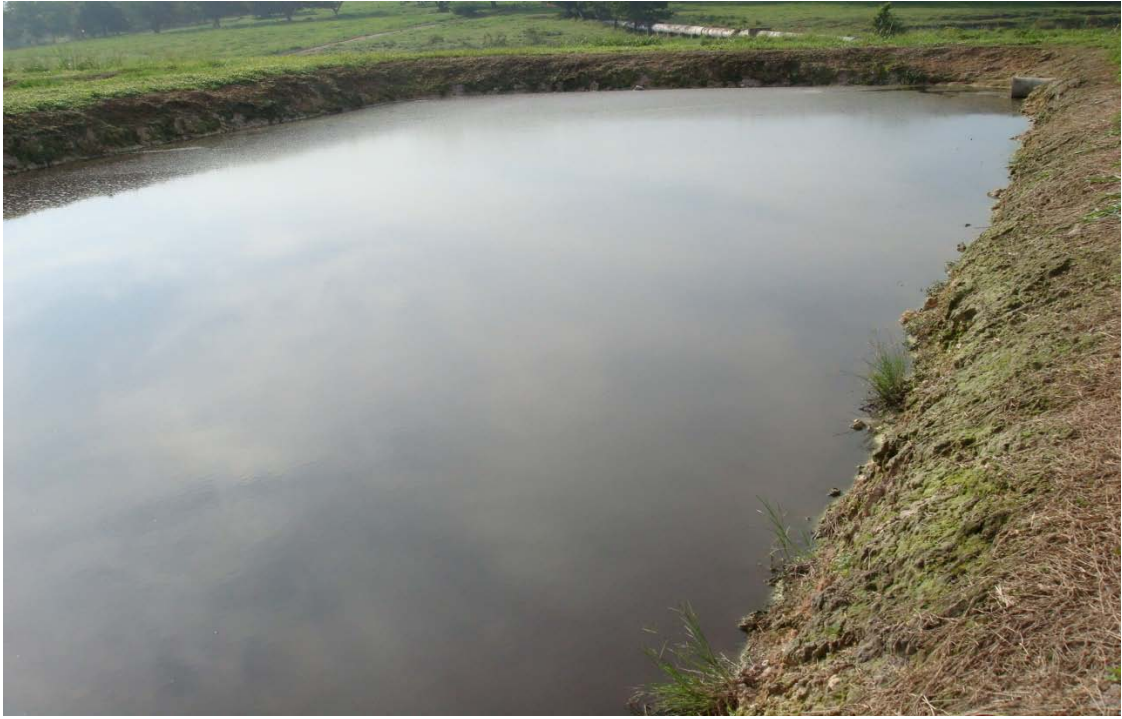
Figure 6.10: The third pond of anaerobic treatment pond before flowing out to sand bed.
