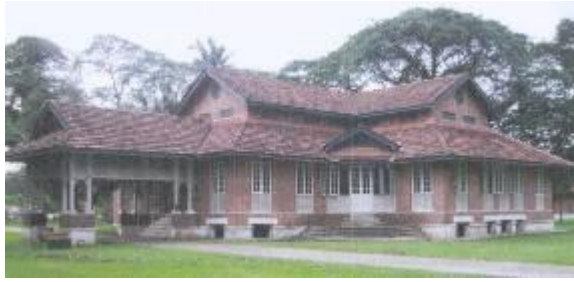
Figure 3.3: Overall view of JKR 1331 Source : UM CORE, 2006
