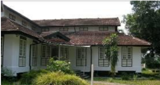
Figure 3.4: Overall view of JKR 1716 Source: UM CORE, 2006
