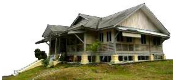
Figure 3.5: Overall view of JKR 541 Source: UM CORE, 2006
