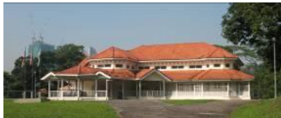
Figure 3.1: JKR 511 main entrance Source: UM CORE, 2006
