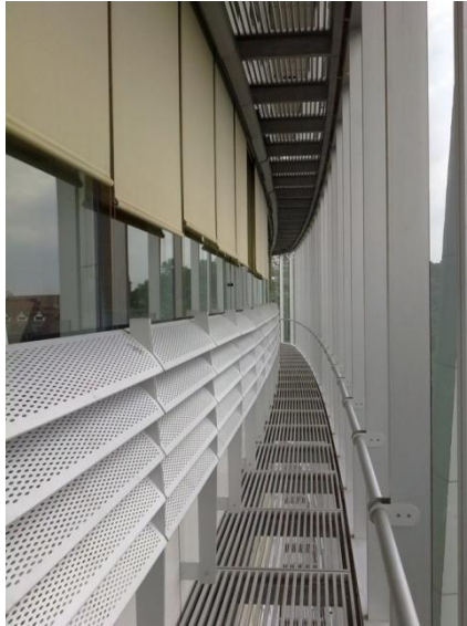
Figure 4.7: The glazing cavity which is a buffer and service route, the shading devices also illustrated
