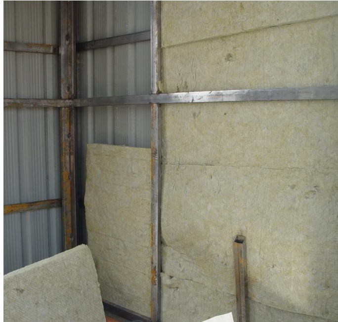
Figure 6.8: A layer of 100mm Rockwool insulation for the wall and internal roof
