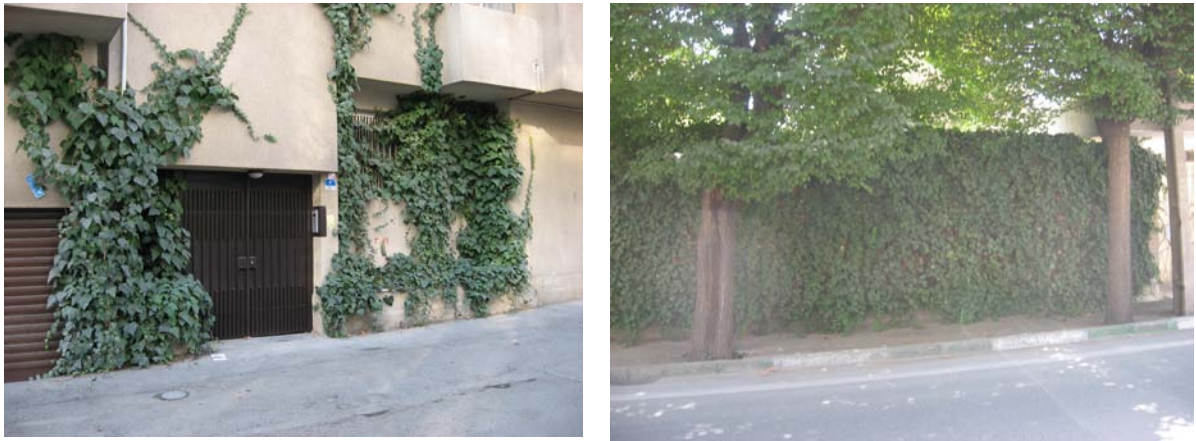
Figure 3.11: Appropriate Design of the boundary walls helps to prevent vandalism and graffiti
