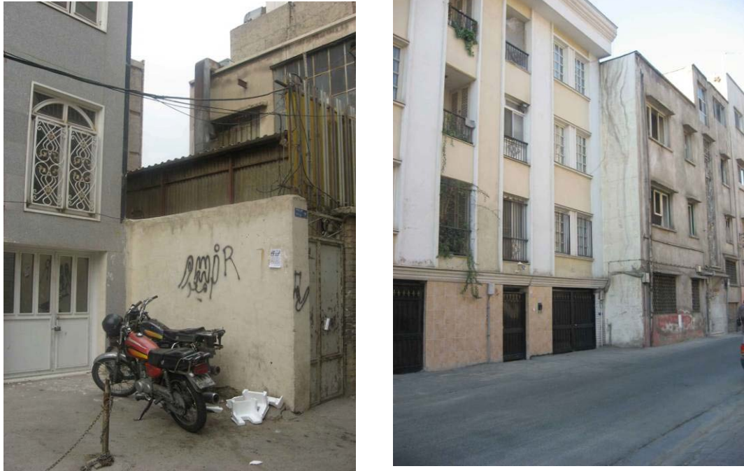
Figure 3.15: The hidden spaces made during the reconstruction of old buildings can give vandals the opportunity to vandalise without being seen
