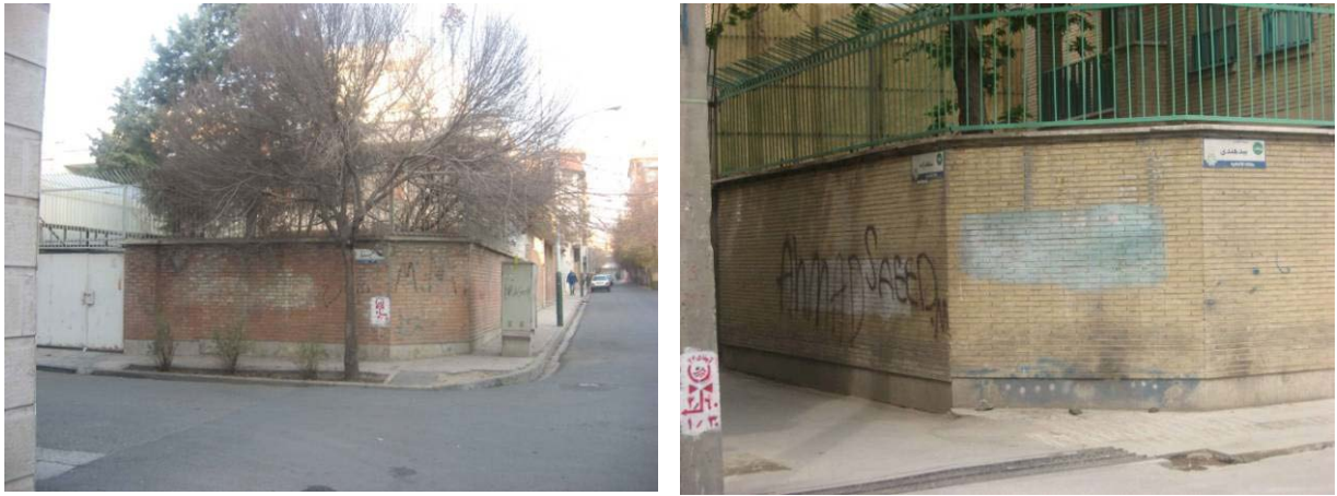
Figure 3.16: Facades vulnerable to vandalism
