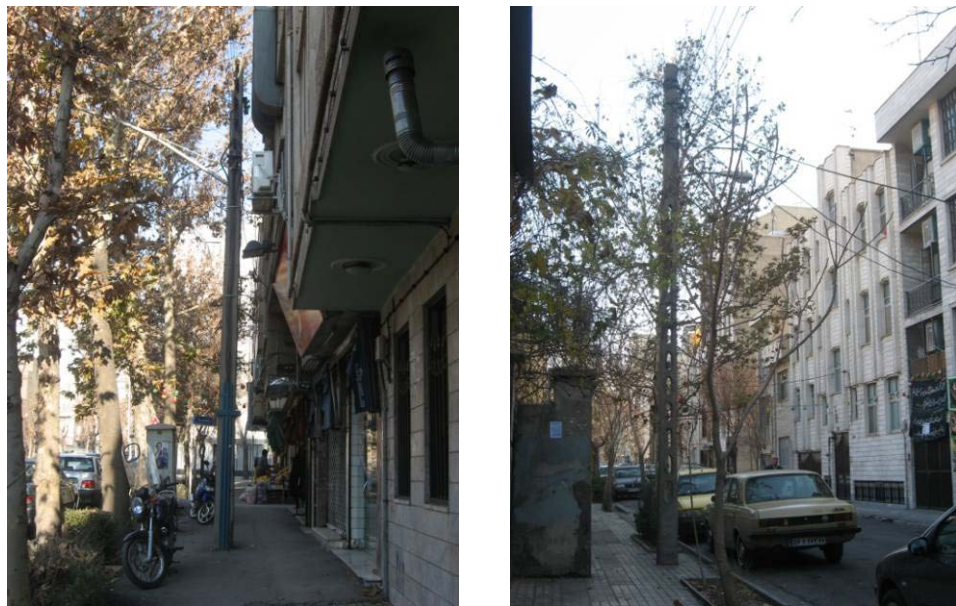
Figure 3.25: Inappropriate pole height can cause safety problems
