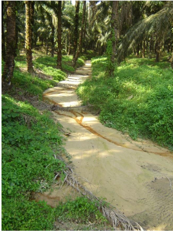
Figure 9.4: Reduction in water way capacity due to sedimentation
