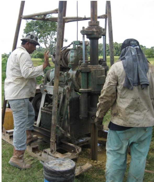
Figure 3.13. Boring equipment to drill a well.
